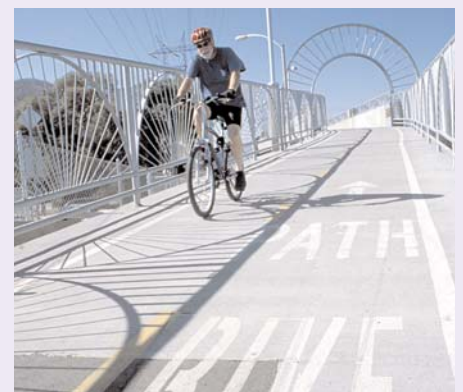
Spanning the Los Angeles River at Los Feliz Boulevard, the Alex Baum Bicycle Bridge is a link in the Los Angeles River Bike Path. One of hundreds of “Call for Projects” transportation projects in part funded by MTA, the bridge opened in May.
