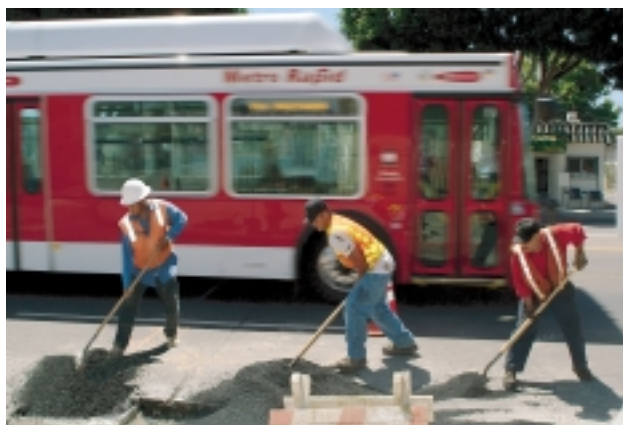
Los Angeles Department of Transportation subcontractors install Metro Rapid signal priority sensors at Florence Avenue and Gramercy Place.
