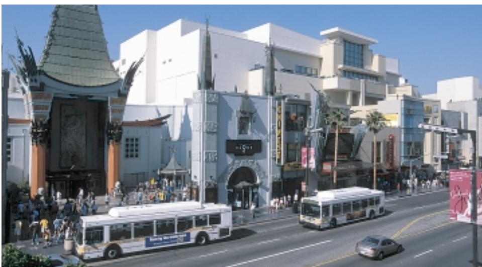
MTA's largest joint development, Hollywood & Highland, is located above the Metro Red Line subway station at the famous intersection. Built next to Grauman's Chinese Theater, the more than 600,000 square foot complex features retail shops, restaurants, general cinemas and the Kodak Theatre, home of the Academy Awards.
