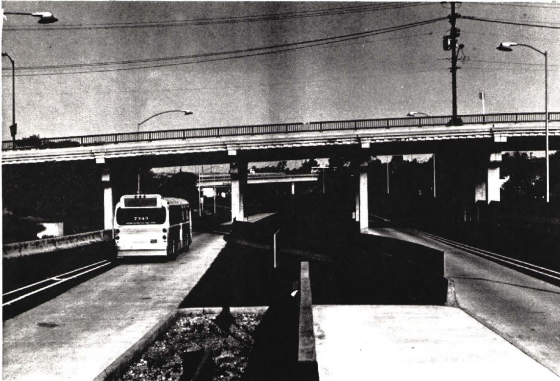
FIGURE 8 LANE CONFIGURATION AT HOSPITAL STATION
