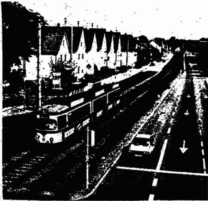
Left: Albtalbahnhof in Karlsruhe. Surface R/W with grade crossing in foreground. Line is between a main highway and local service road accessing the residential area at left.
