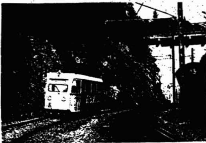
Below: Oslo tramway line in rock cut. Four-axle "Goldfish Car." (Note gauntlet track at right.)
