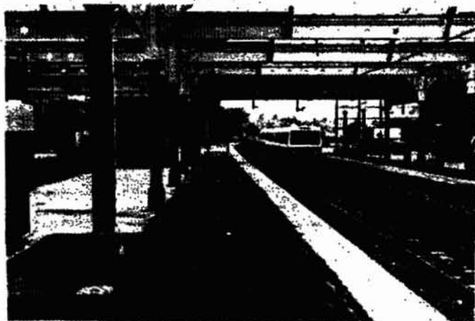
Left: Whitley Bay. Existing structure was in good condition, and simply required repainting.
