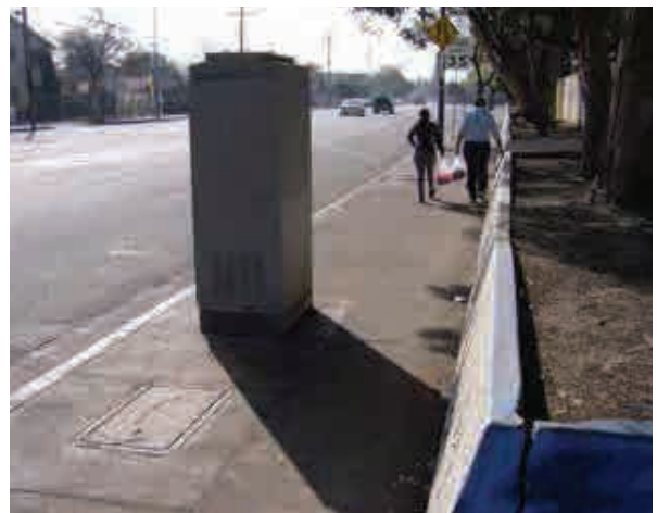
3.1 Utility obstructions in sidewalk right-of-way
