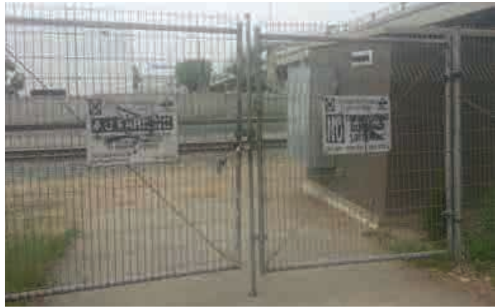
1.7 Unclear Safety Signage
