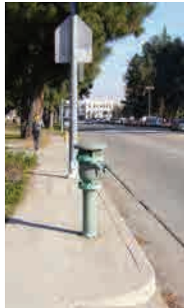
3.1 Utilities in sidewalks
