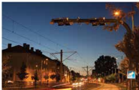
Over road cantilever (Sweden)
