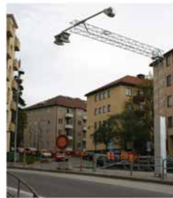
Over road cantilever (Sweden)
