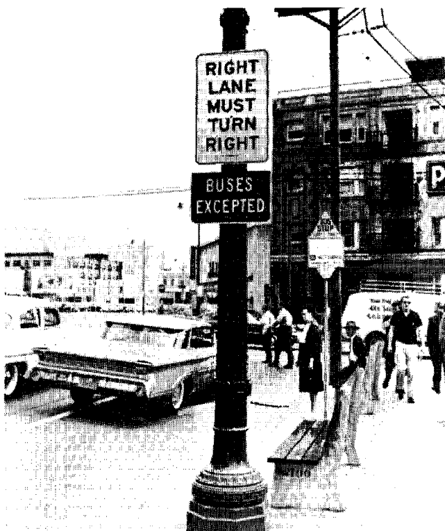
Photo at left represents Bus Stop with Right Turn Exemption.
