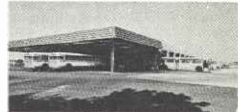
2. MAINTENANCE BUILDING (View Looking Northwest)
