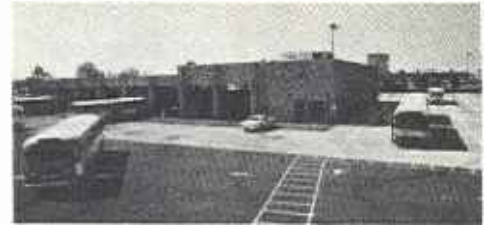
1. MAINTENANCE BUILDING (View Looking West)
