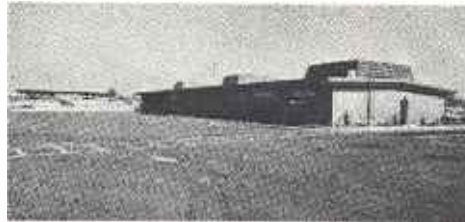
3. TRANSPORTATION BUILDING (View Looking Northeast)
