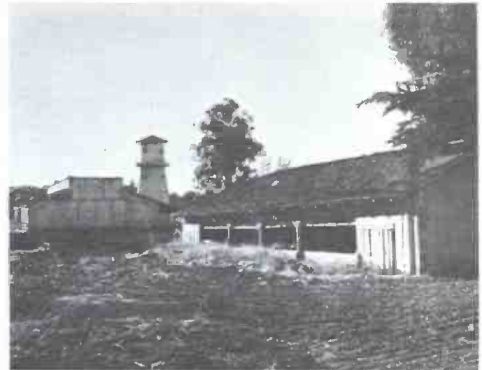
Farm Structures Located on Bayly Ranch, Adjacent to Proposed Project Site.
