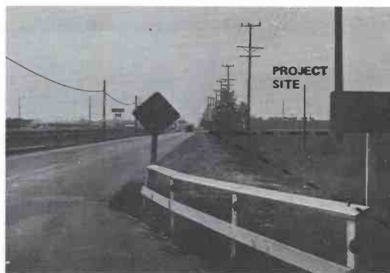
Canoga Avenue narrowing to one lane both directions, with industrial uses in the background and the site to the right (view south)
