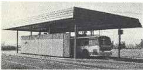
4. BUS WASHER FACILITY (View Looking Northwest)
