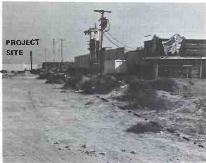
Eastern and Southern Boundaries of Project, from Corbin Ave. (View East).
