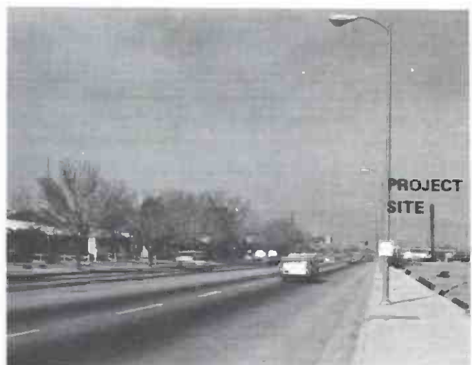
Corbin Ave., Vicinity of Intersection of Corbin Ave. and Nordhoff St. (View North).
