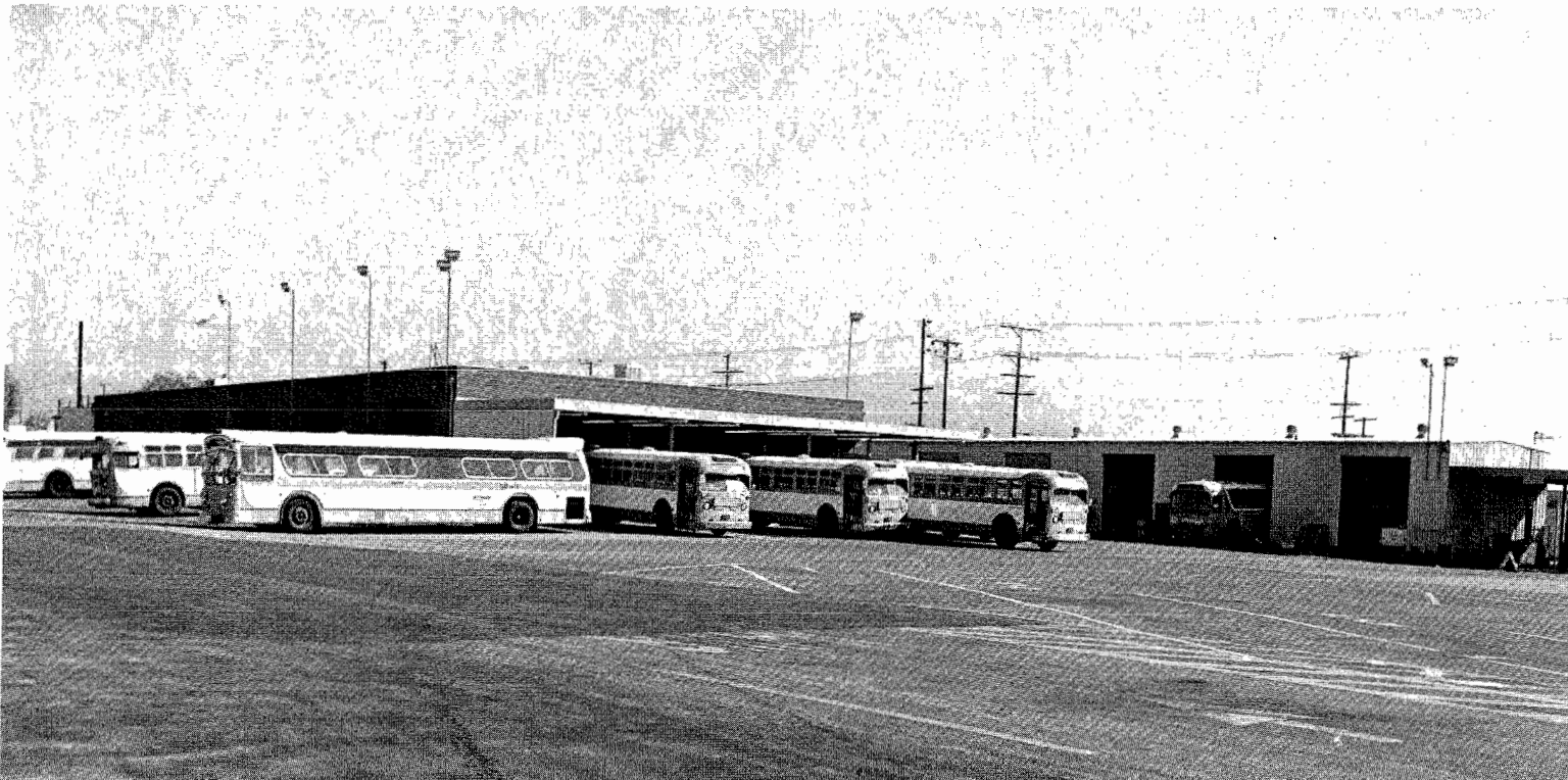
Bus operating yard in Sun Valley, California.
