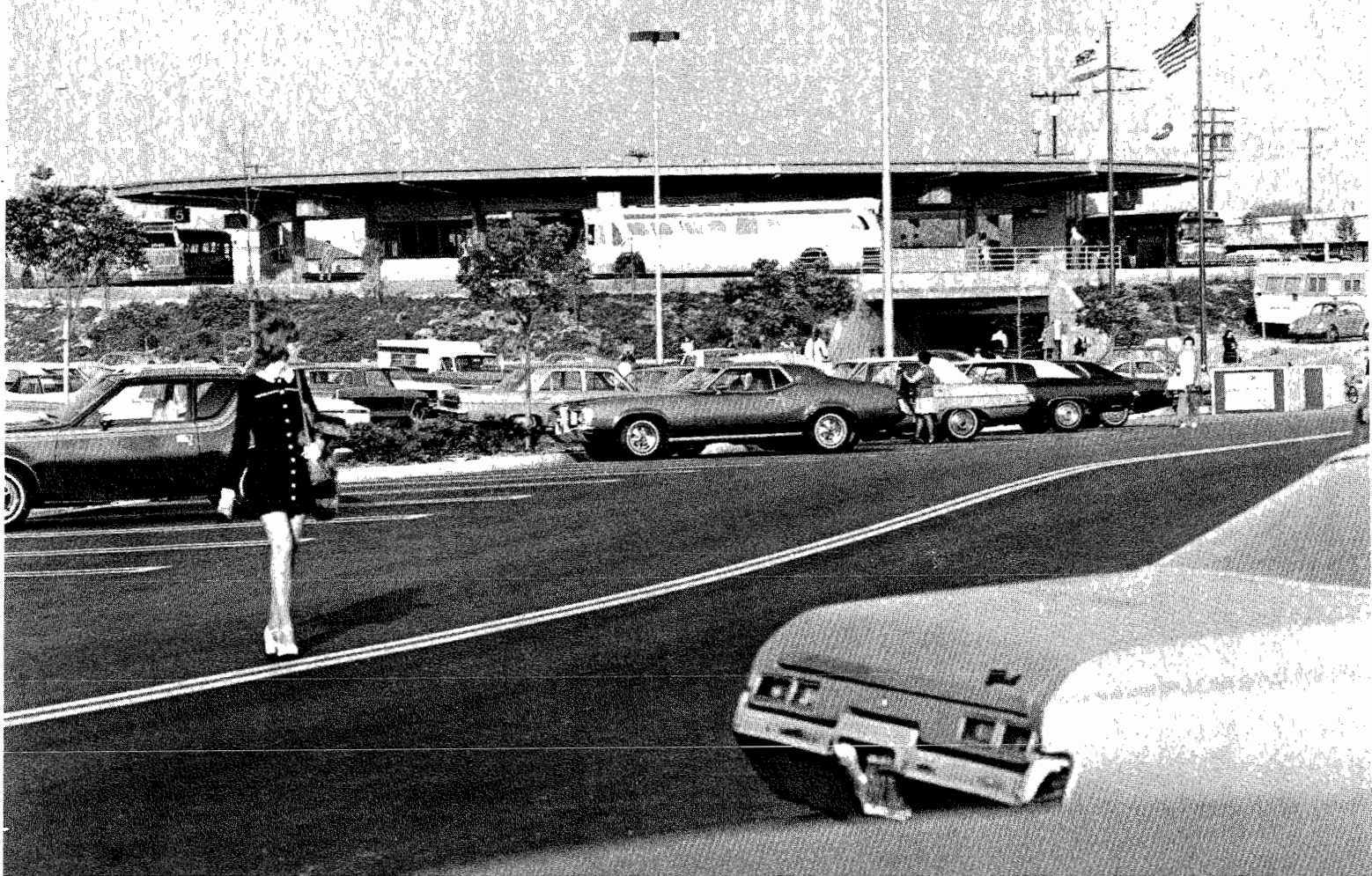
Modern bus passenger station serving the Busway lane of the San Bernardino Freeway at El Monte, California.
