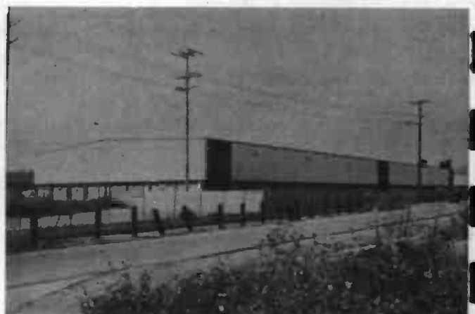
Northwest Site Area, Looking Northwest At Eureka Metals Co. & Rail Spur Tracks.
