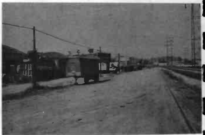
Northeast Site Area, Looking North At Rear Of Calusa & Metalex Companies, Santa Fe Main Trackline At Right.
