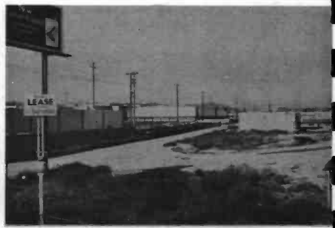
Southcentral Site Area, Looking North From Macy St., SAE Electronics At Left.
