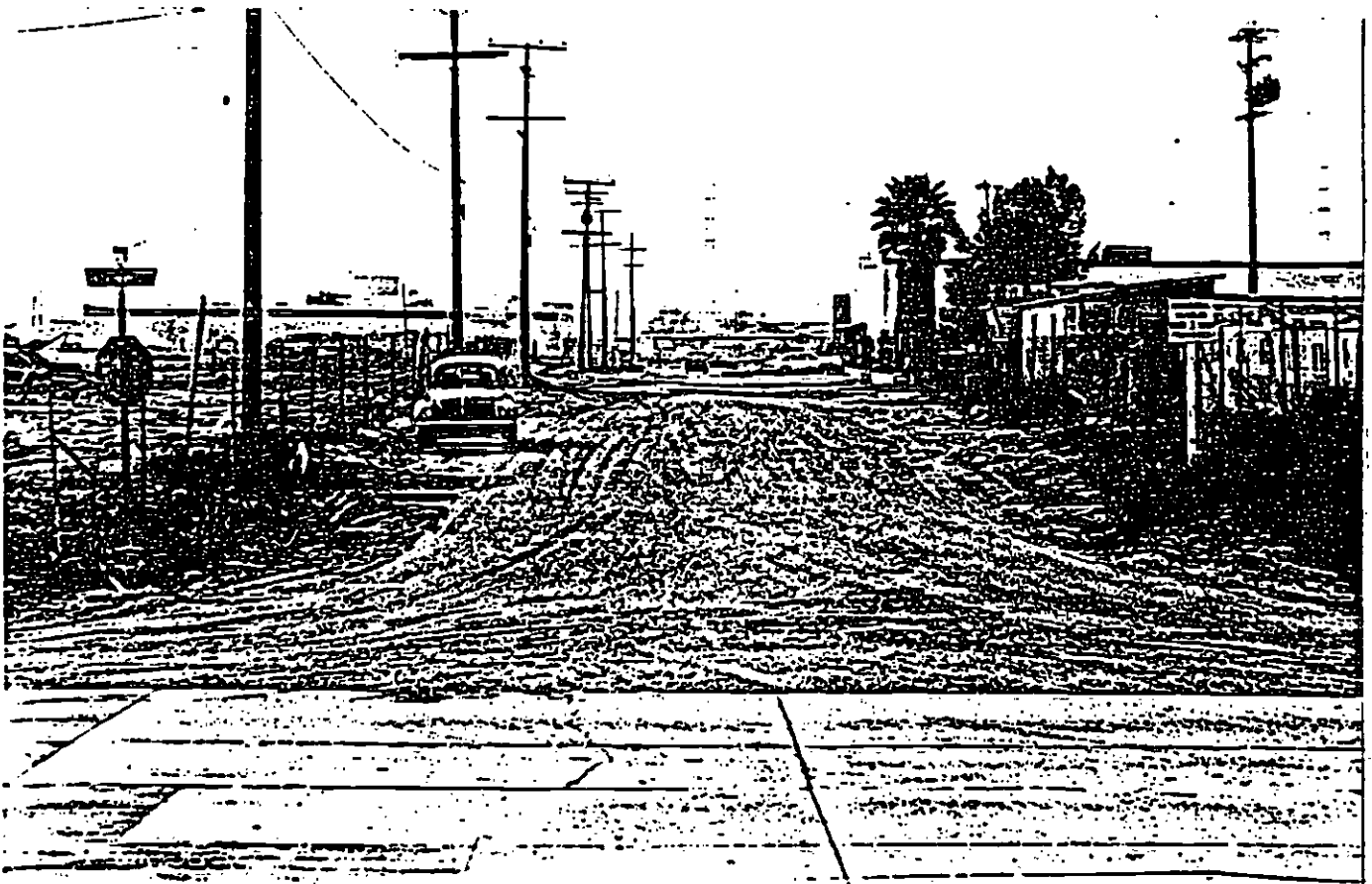
PHOTO D - LOOKING WEST ON GRIFFITH ST. SITE IS LOCATED TO LEFT.
