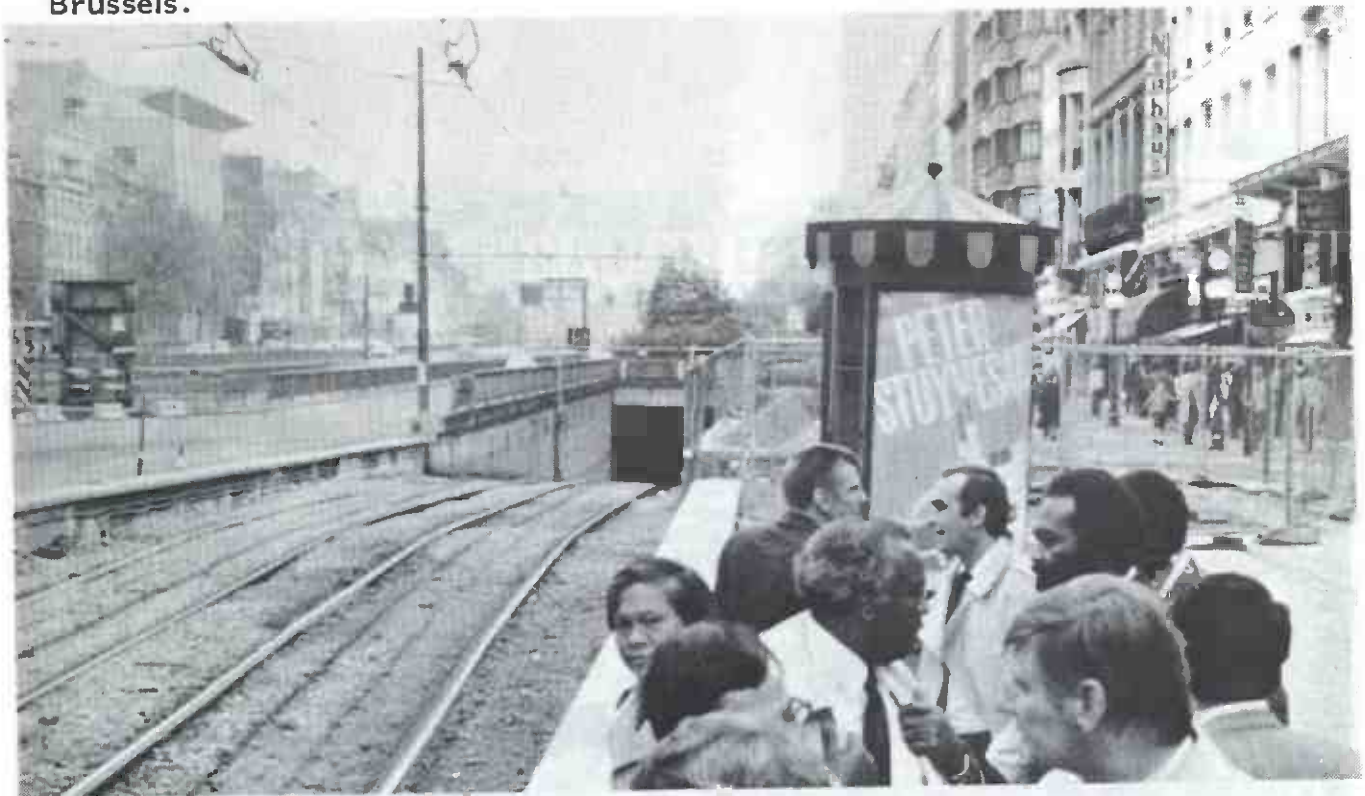
"Pre-metro" is one system that operates in subway as a heavy rail-type operation (above) and on the surface in a light rail mode (below). It has proven to be a successful concept in transforming public transit in Brussels.
