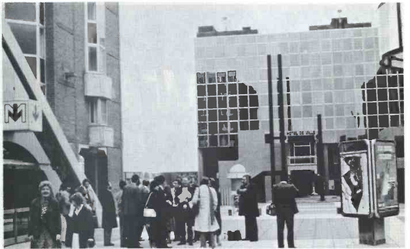
VAL was designed to minimize capital and operational costs. But the planners did take advantage of incorporating the system in commercial/residential areas as seen in this station plaza level. A hotel is located in the background. Apartments at left and retail business can be seen.
