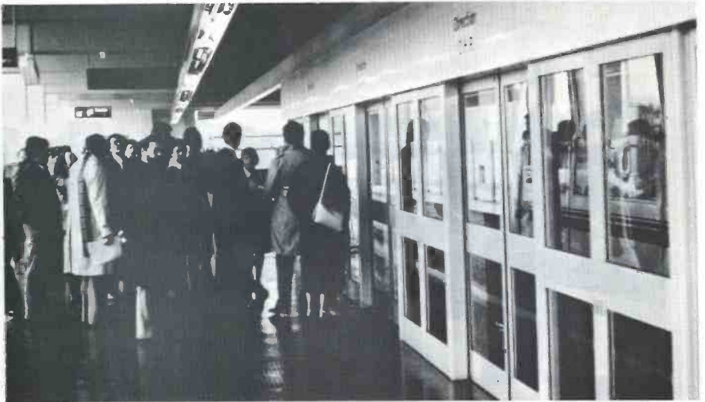
Automatic glass doors open and close to allow patrons to ride the VAL system when trains enter and exit stations. The doors serve as a protective barrier for patrons, too.
