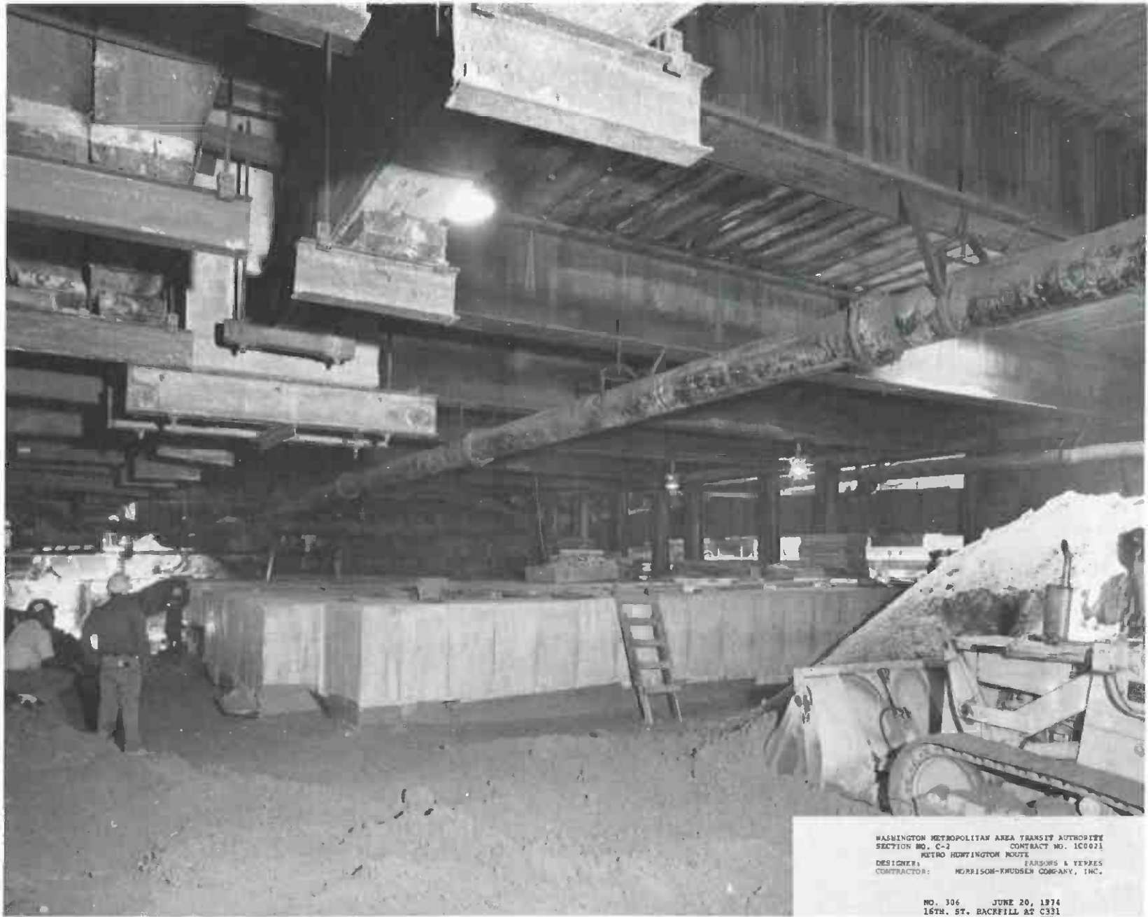
FIGURE 12 PIPES AND CONDUITS SUPPORTED BY HANGERS ATTACHED TO STREET DECKING
