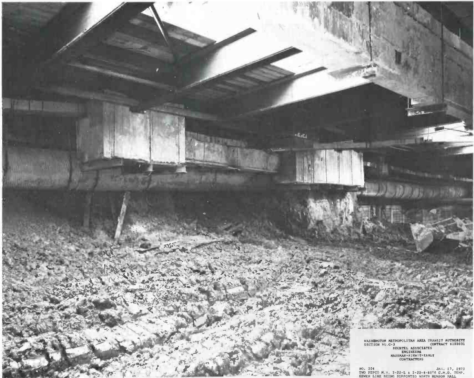
FIGURE 13 TEMPORARY METAL PIPE SUPPORTING STORM DRAINAGE; CAST-IN-PLACE CONCRETE MANHOLES AND CONCRETE ENCASED DUCTS ARE SUPPORTED IN PLACE
