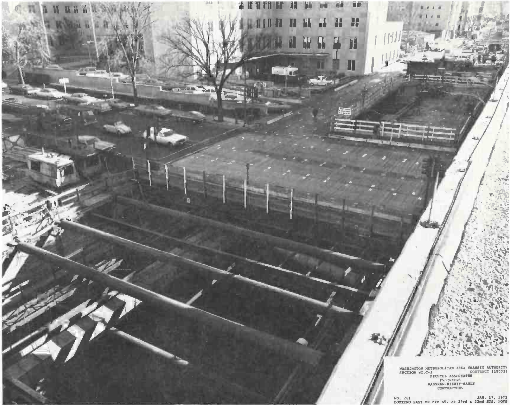
FIGURE 7 DECKED STREET WITH TEMPORARY SIGNALS
