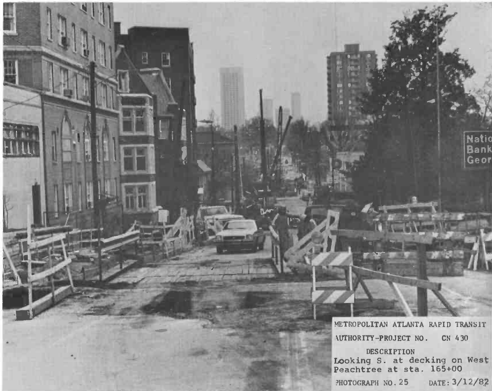
FIGURE 8 DECKING SERVES AS TEMPORARY ROADWAY AND STAGING AREA FOR CONTRACTOR'S EQUIPMENT AND MATERIALS
