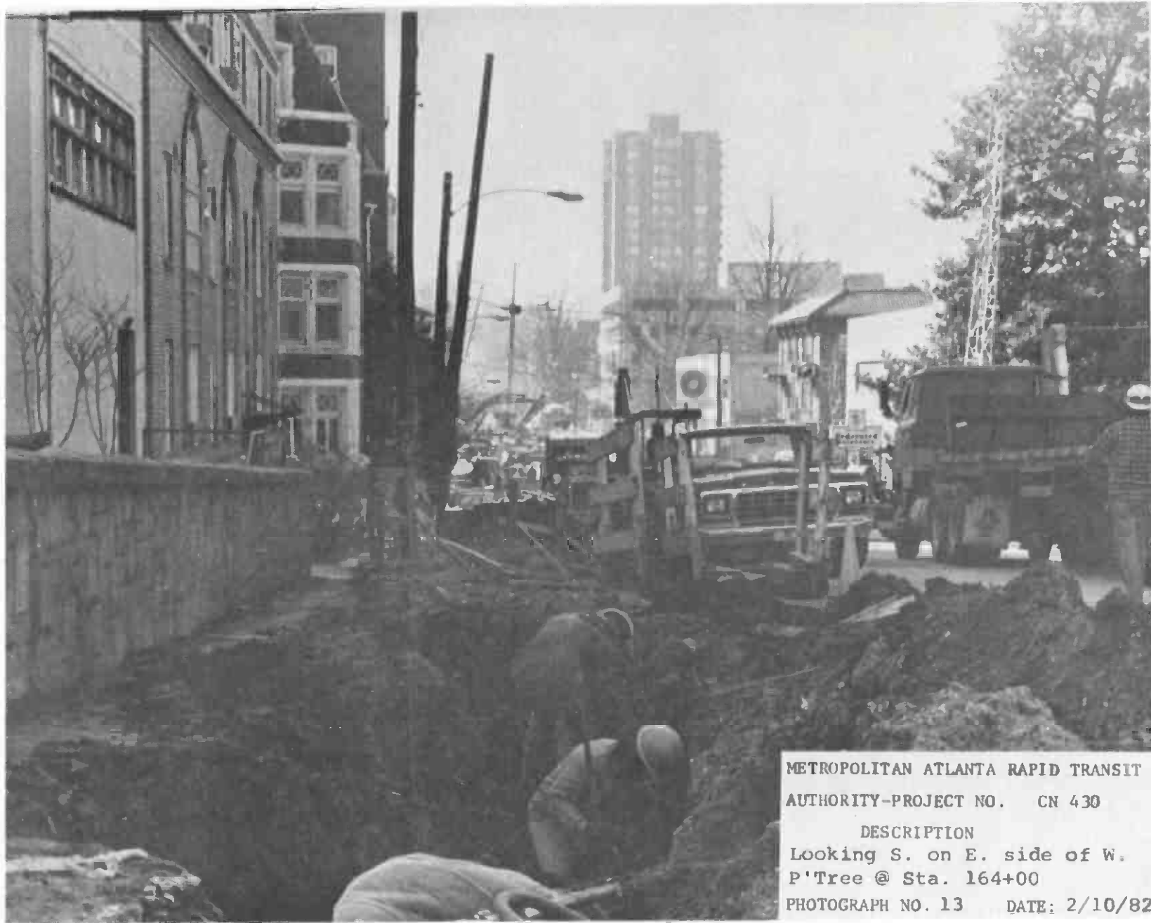
FIGURE 3 LOCATING AND REARRANGING UTILITIES AT THE CONSTRUCTION SITE
