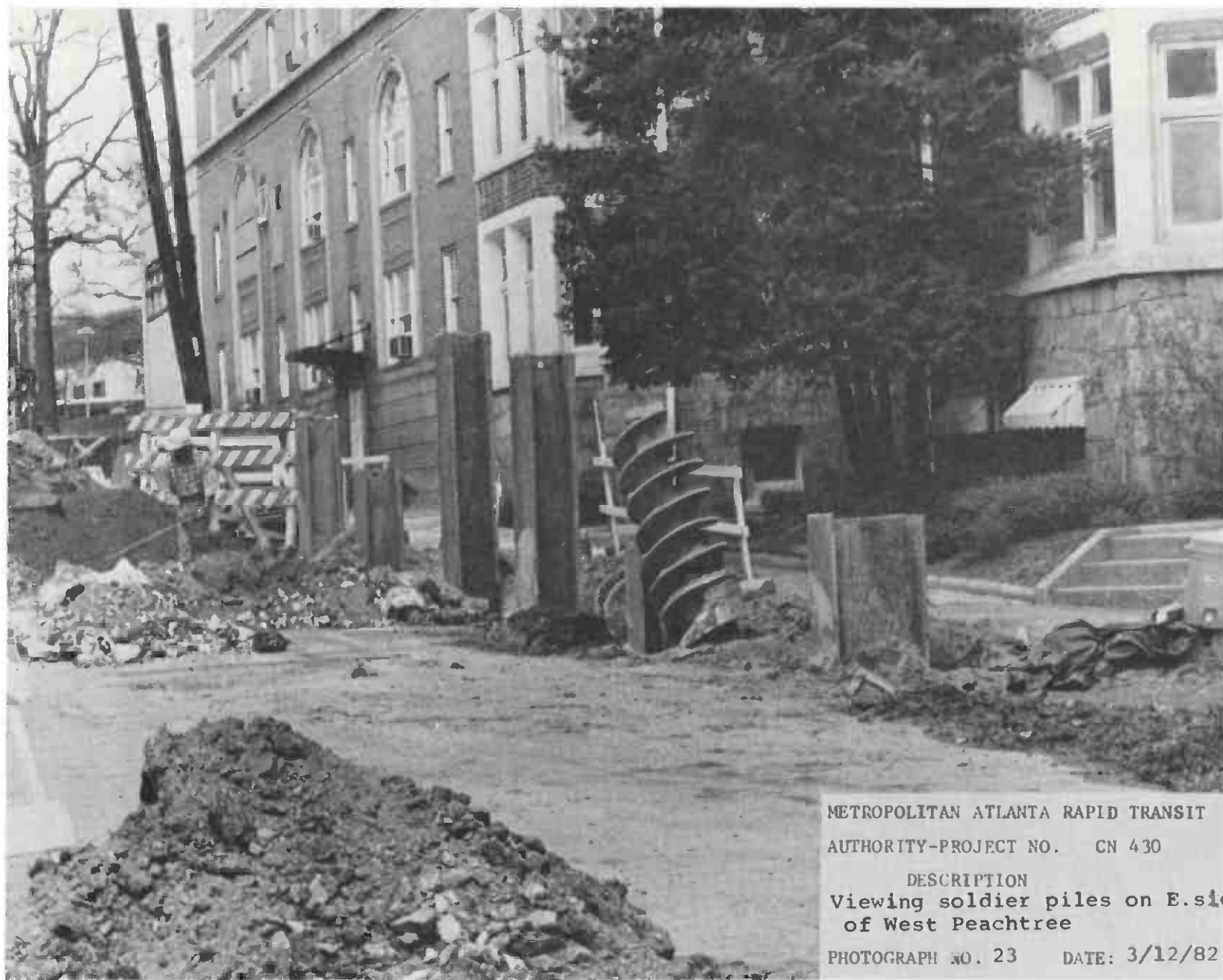
FIGURE 4 SOLDIER PILES AROUND FUTURE STATION PERIMETER
