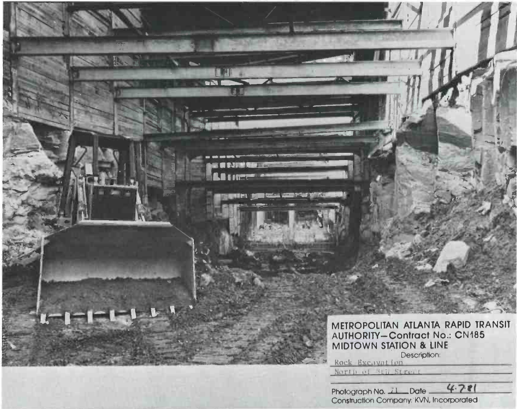
FIGURE 18 EXCAVATION BENEATH THE DECKING WITH HEAVY EARTH-MOVING EQUIPMENT
