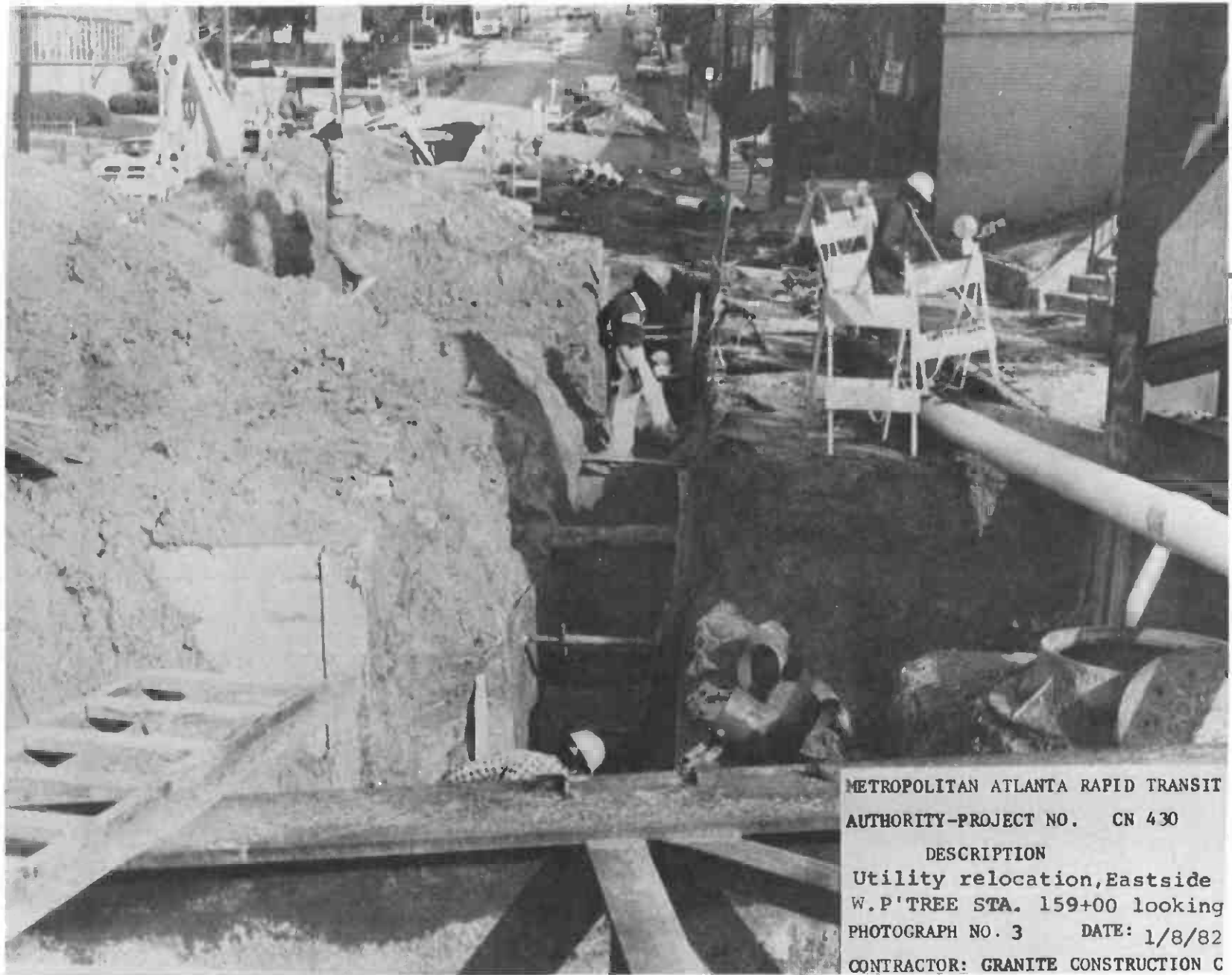
FIGURE 5 SPACE BETWEEN SOLDIER PILES AND EXISTING BUILDING IS USED FOR REARRANGEMENT OF UTILITIES
