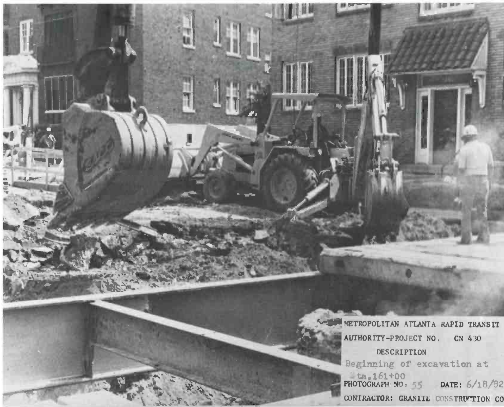
FIGURE 6 DECKING PREPARATION: REMOVAL OF STREET PAVEMENT AND INSTALLATION OF STEEL BEAMS
