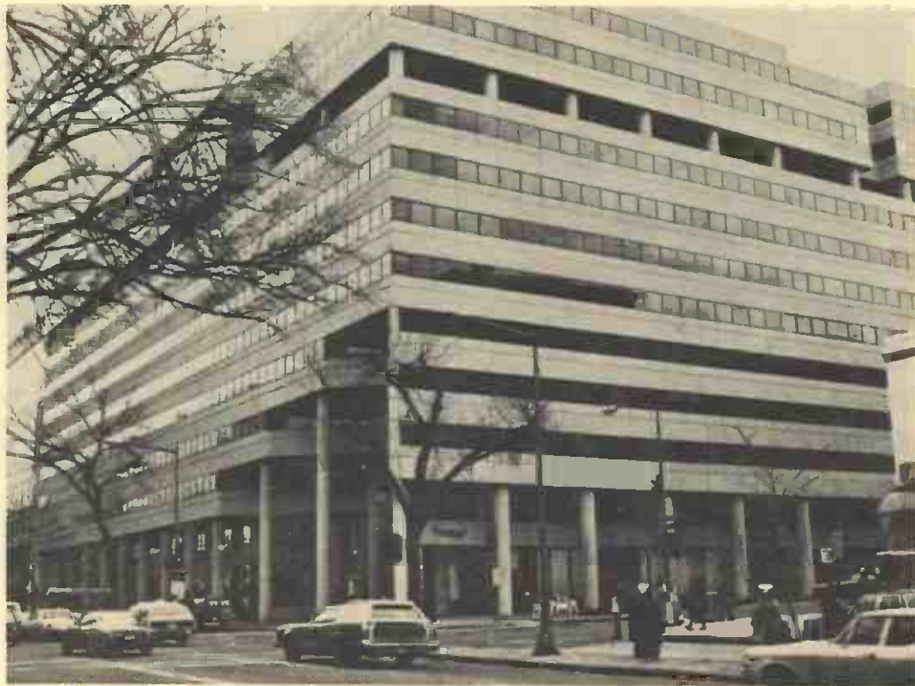
11 A joint development example from Washington, D.C., International Square, shows how the building's footprint was "notched out" at the lower floors to provide ample room for the integration of the portal without any loss of leasable air rights above.
