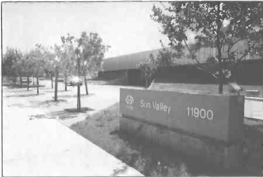
ADMINISTRATION BUILDING ENTRANCE AT DIVISION 15
