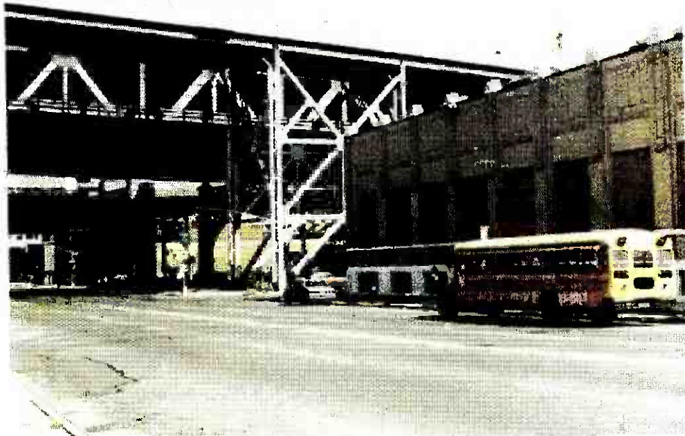
SILVERCUP RECORDING STUDIOS, ADJACENT TO QUEENSBORO BRIDGE, NEW YORK CITY.
