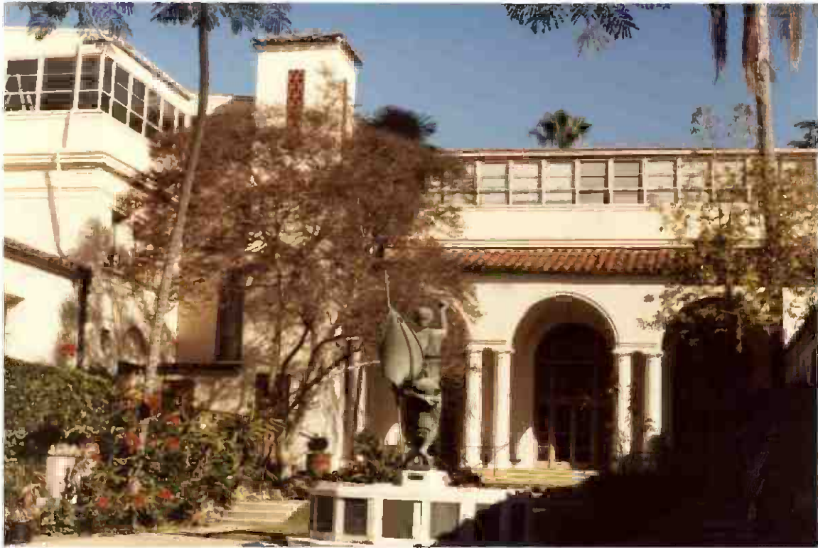
THE EBELL CLUB OF LOS ANGELES BUILDING AND WINDSOR SQUARE THEATER 4400 WILSHIRE BOULEVARD, LOS ANGELES
