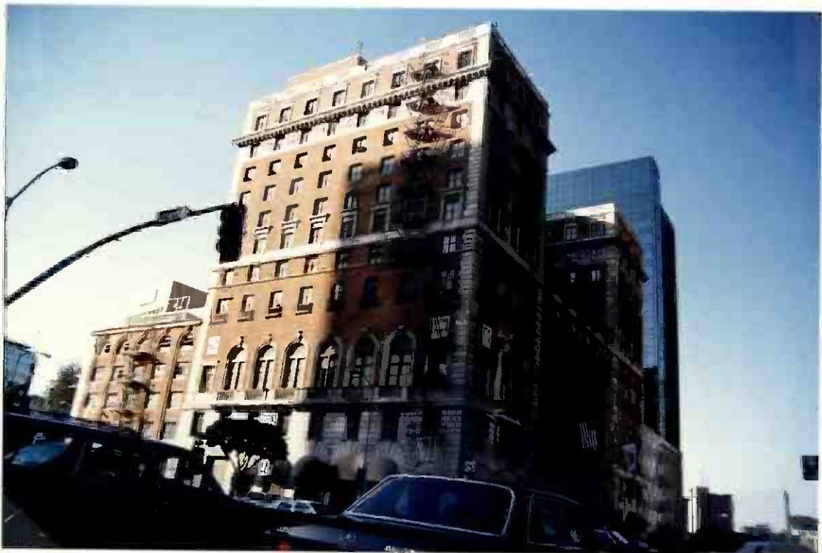
Jonathan Club- 545 South Figueroa Street- Built 1924
