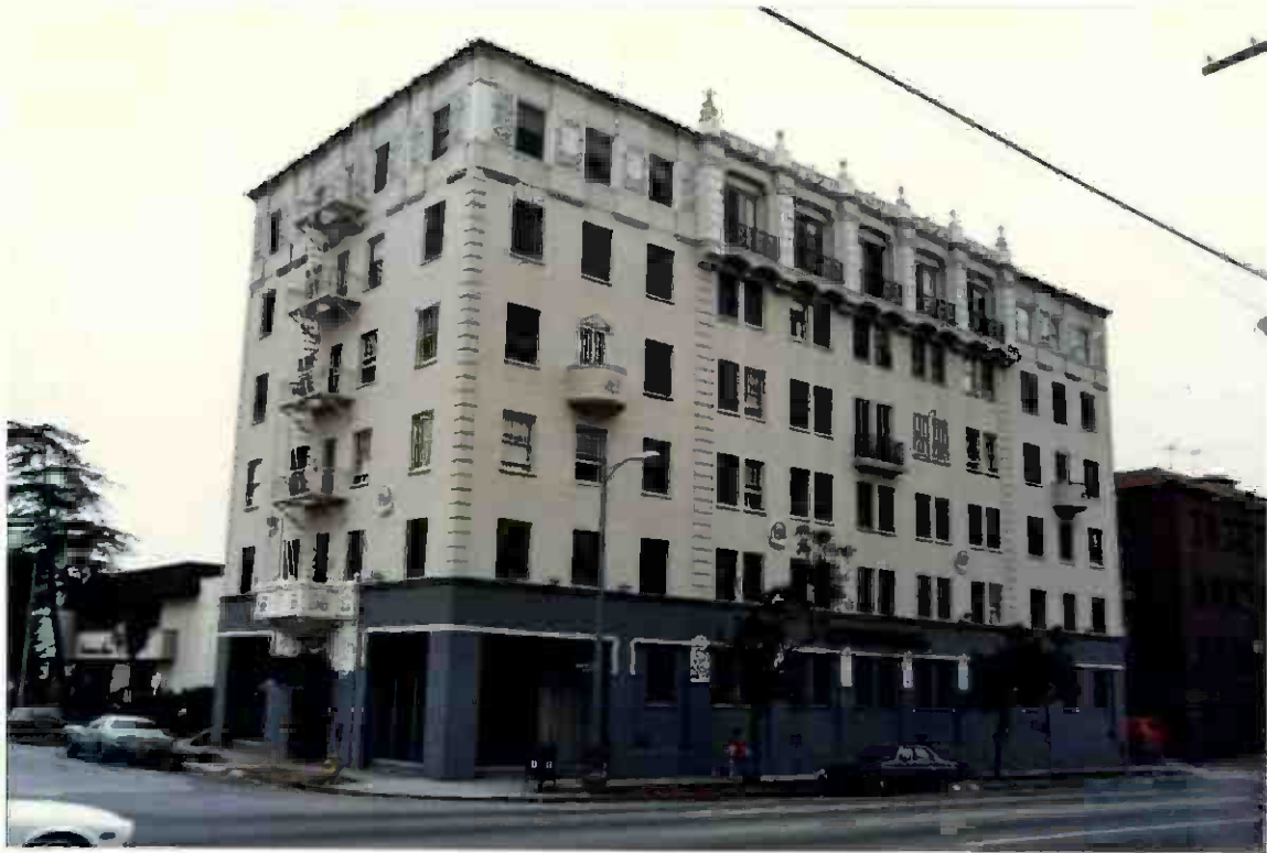
Apartments- 801 South Gramercy Drive- Built 1926
