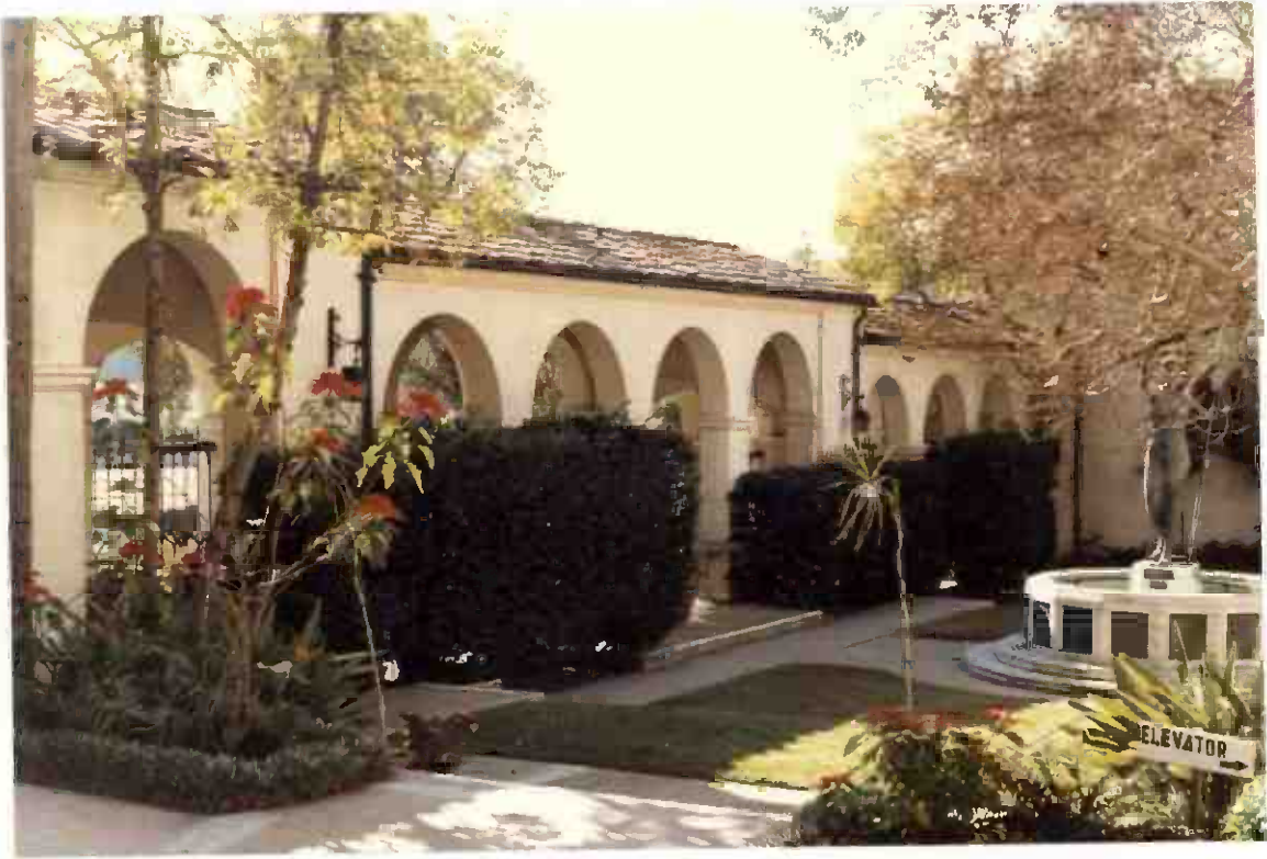
THE EBELL CLUB OF LOS ANGELES BUILDING AND WINDSOR SQUARE THEATER 4400 WILSHIRE BOULEVARD, LOS ANGELES
