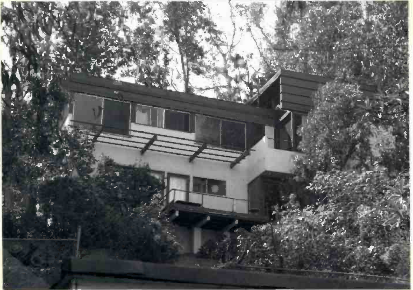
John De Keyser Duplex 1911 North Highland Avenue
