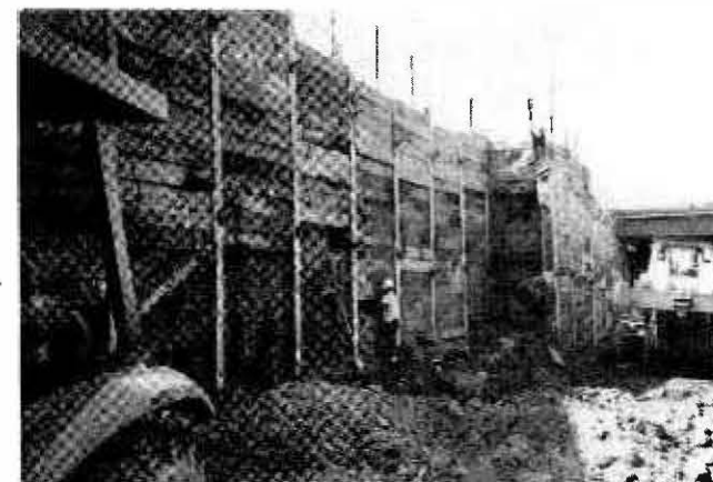
LAGGING INSTALLATION ON SOUTH WALL OF EXCAVATION SUPPORT SYSTEM
