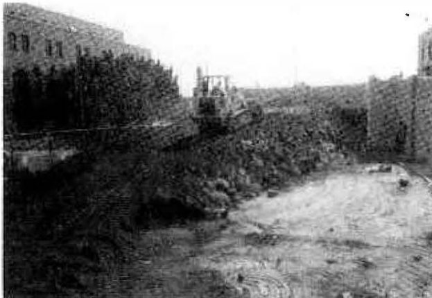
CONSTRUCTING TEMPORARY MACY STREET RAMP AT UNION STATION
