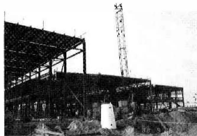
NORTH END OF BUILDING
