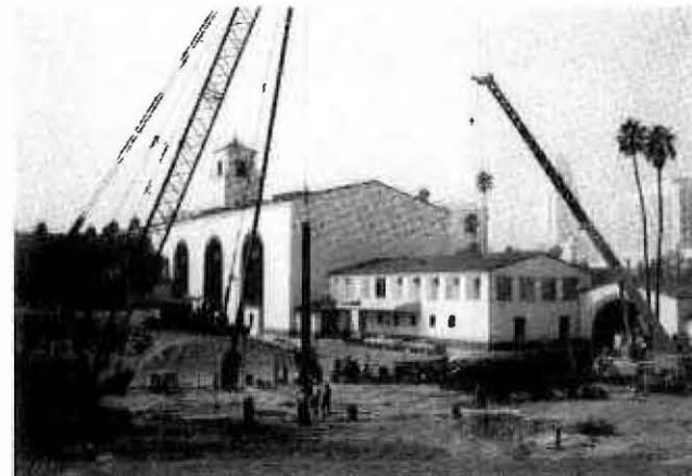
INSTALLING SOLDIER PILES FOR THE SHAFT AT UNION STATION
