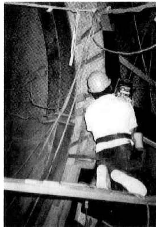
AL TUNNEL HDPE INSTALLATION SUMP STRUCTURE
