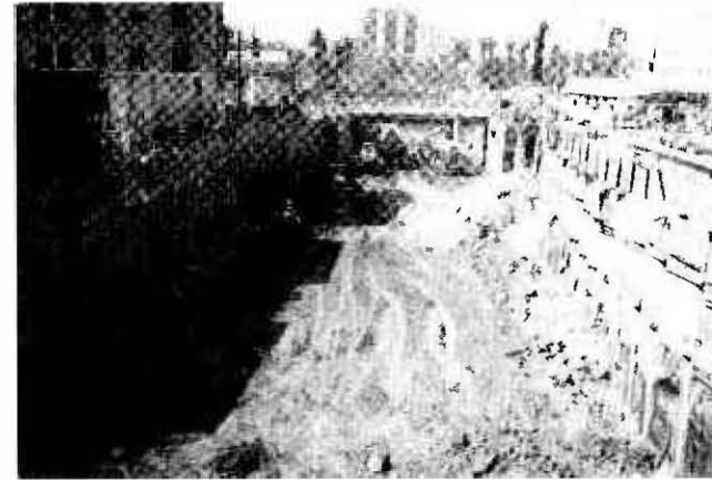
STATION EXCAVATION, EAST OF WESTLAKE AVE. ADJACENT TO A171 CONTRACT
