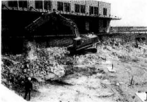
DEMOLITION OF PORTION OF REA BUILDING AT UNION STATION SHAFT
