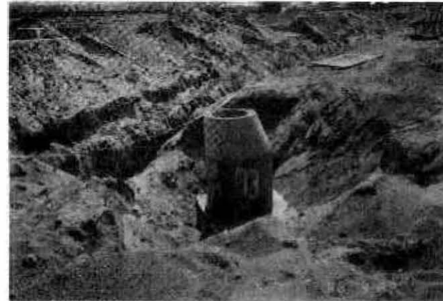
STORM DRAIN MANHOLE INSTALLATION
