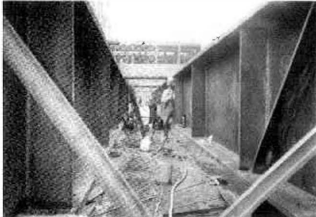
36" DECK BEAMS UNDER FABRICATION WITH THE WELDING OF STIFFENERS
