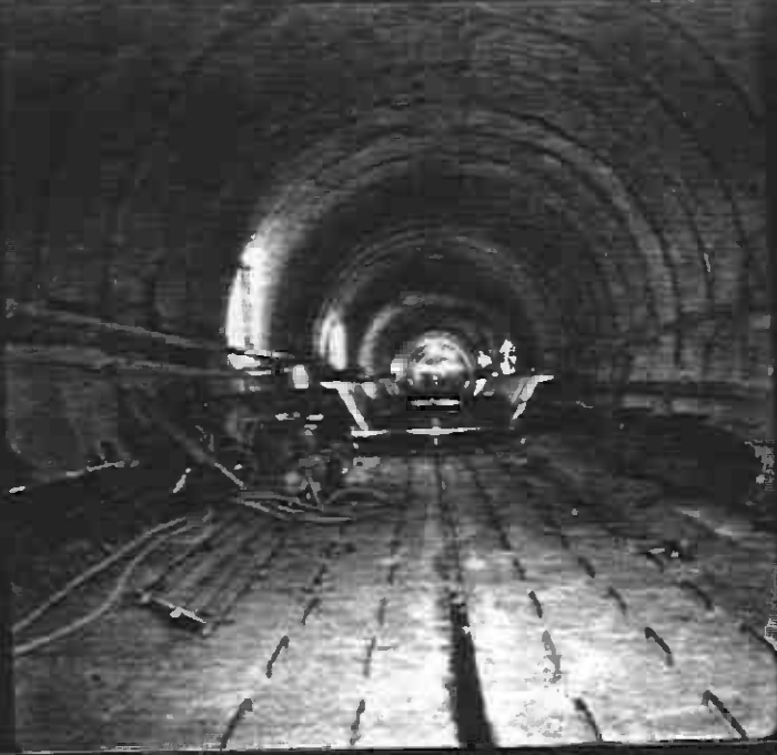
SLIDE A171-35 AL tunnel invert concrete (view facing west) (1/89)
