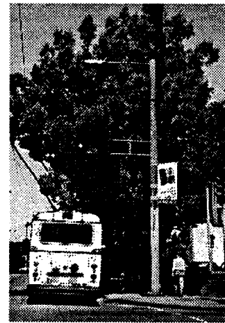
Fig. 3.3-27: ETB pole, bracket arm and trolley wires partly obscured by tree canopy at intersection
