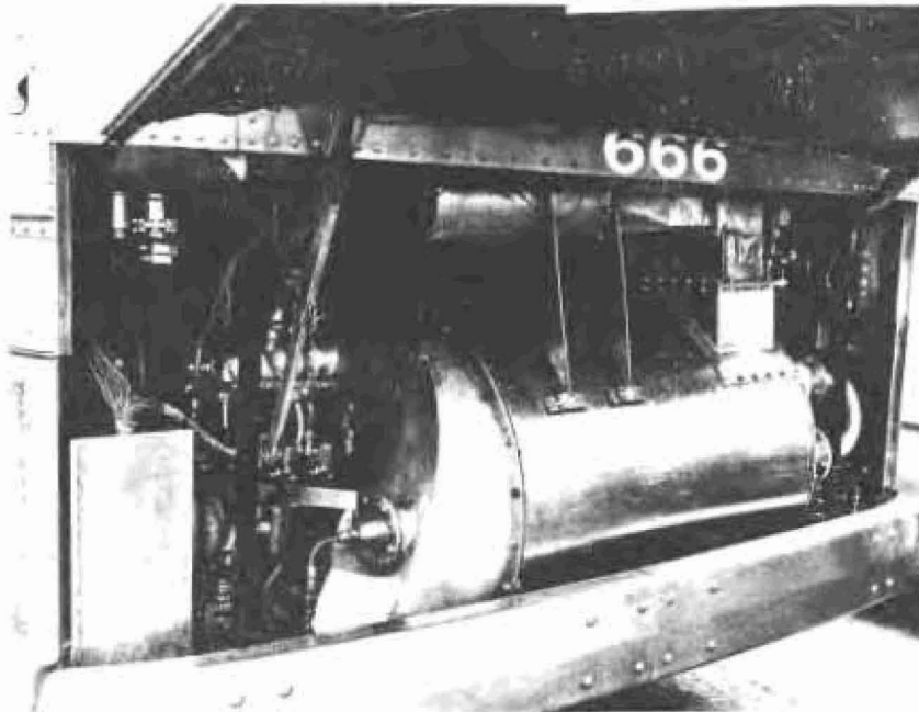
Figure 1. Installation of Boiler in William Brobeck & Associates Demonstration Bus.
