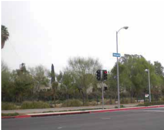
3.7 Orange Line multi-use trail without accessible ramp
