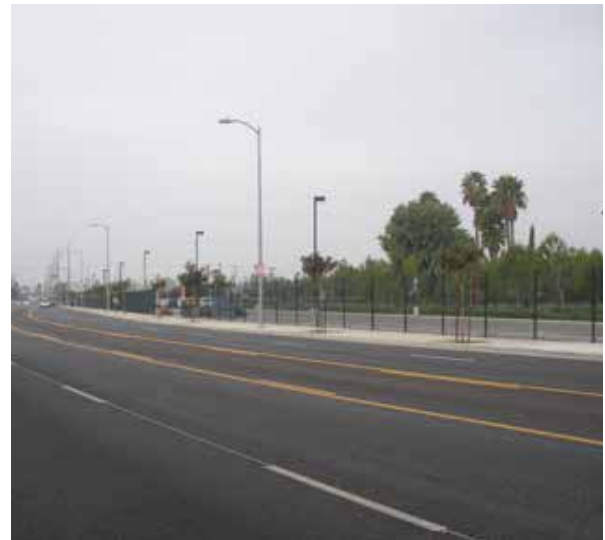
3.8 Looking across Oxnard to fenced and underutilized Metro park-and-ride lot
