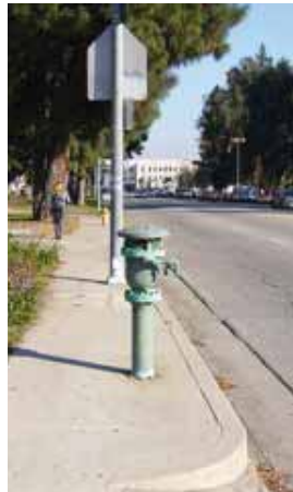
3.1 Utilities in sidewalks
