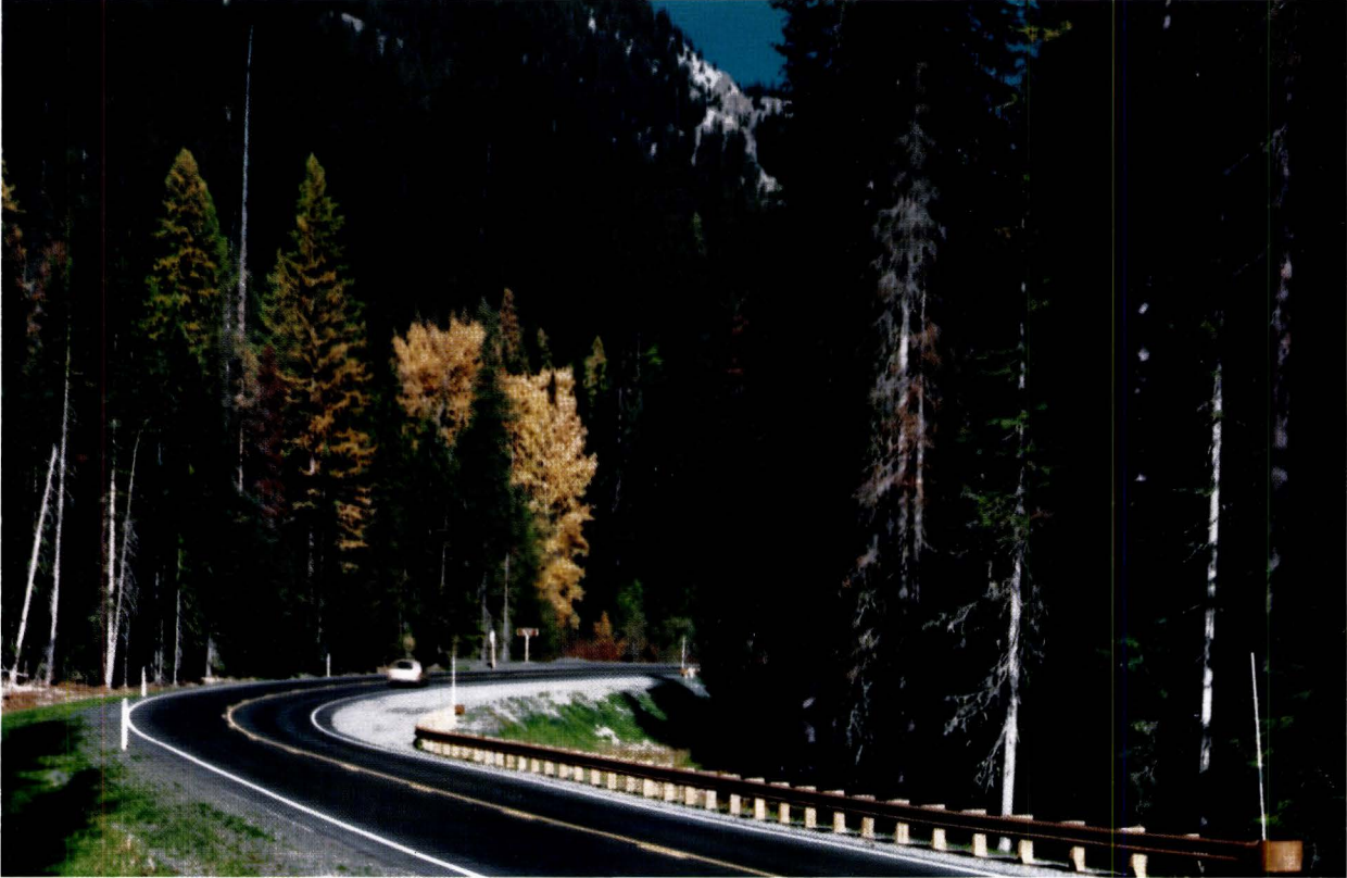
SR 410 in Mt. Rainier National Park, Washington, presents a typical two-lane scenic road built through a partnership arrangement between Federal and State agencies. The byway is blended into pristine scenery making possible an enjoyable and relaxing experience for the recreation seeker.
