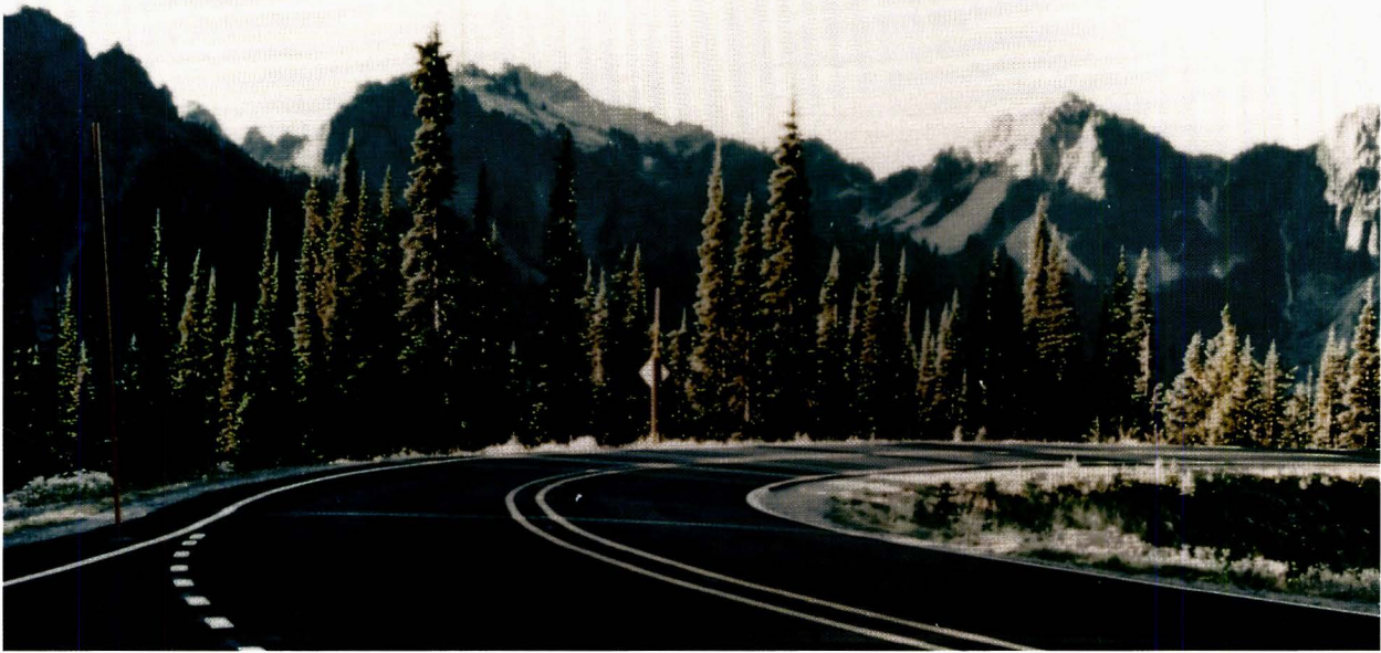
The Nisqually Paradise Road in Mt. Rainier National Park, about 80 miles southeast of Seattle, Washington. This scenic road would be an example of a potential candidate, along with others, for recognition as an “All-American Road.” This recognition effort would be a joint Federal-State-local-private sector effort.
