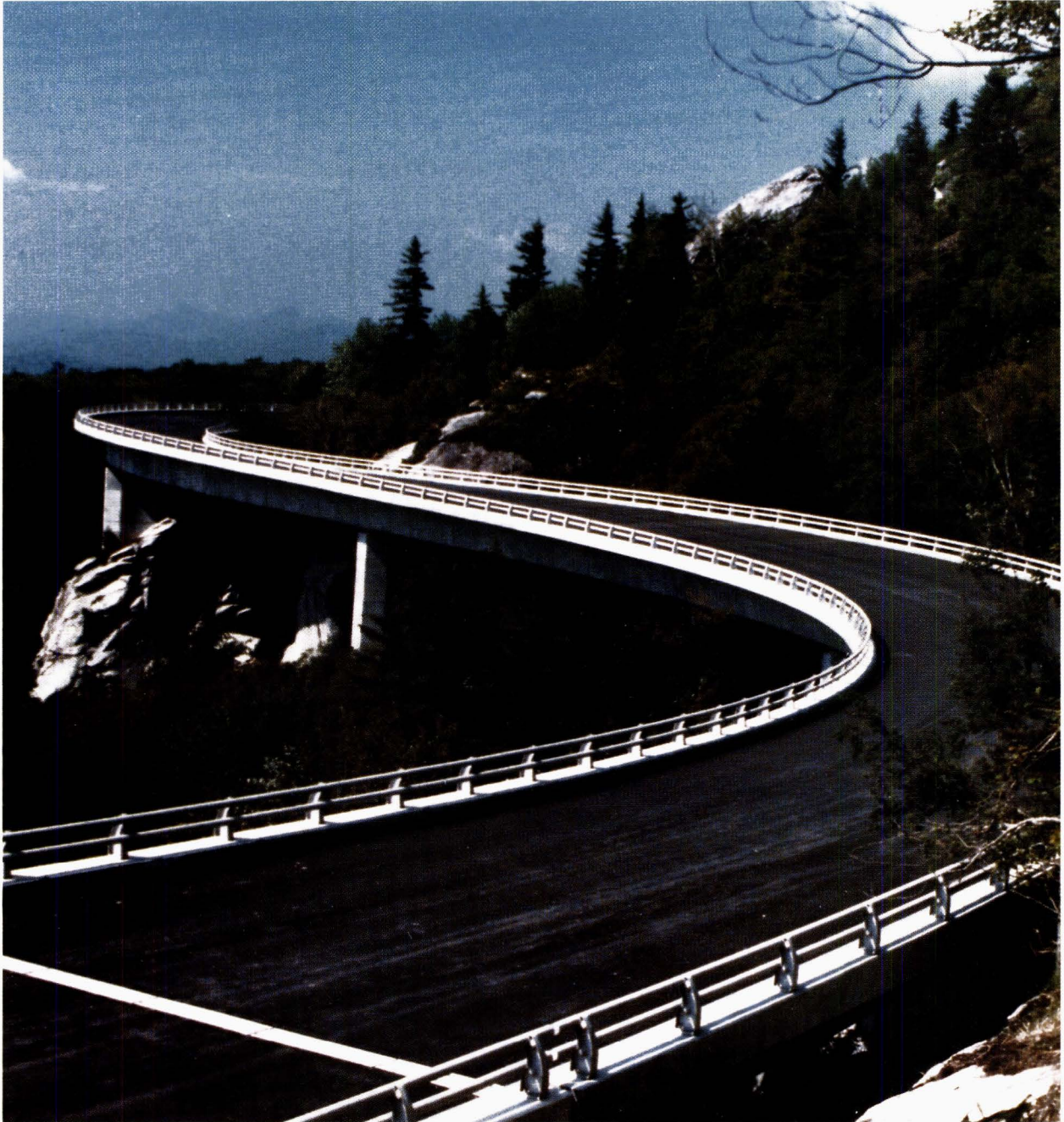
The Linn Cove Viaduct on the magnificent Blue Ridge Parkway in North Carolina. This facility represents the embodiment of many of the elements identified in this report.
