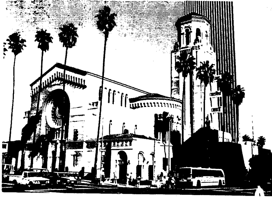
SOUTH AND WEST ELEVATIONS OF BUILDING (LOOKING TO NORTHEAST)
