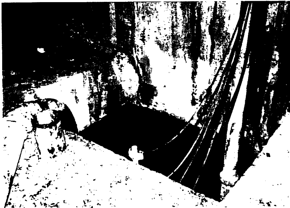
SUMP PIT IN VENTILATION SHAFT NORTHWEST CORNER OF BUILDING
