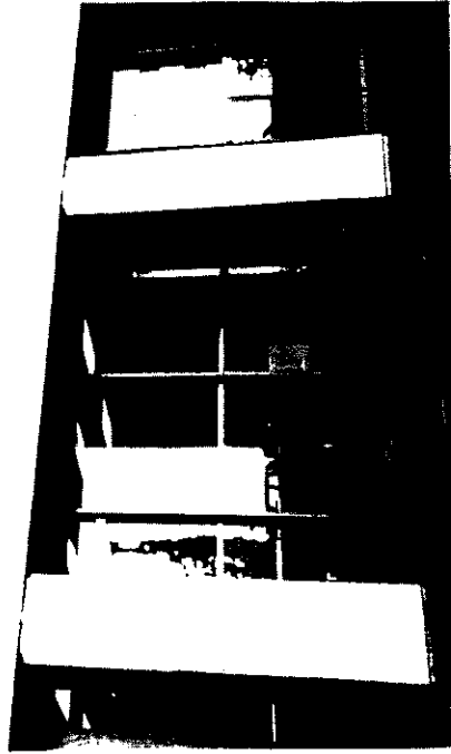
INTEGRAL FRAME/FACADE OF CAST CONCRETE
