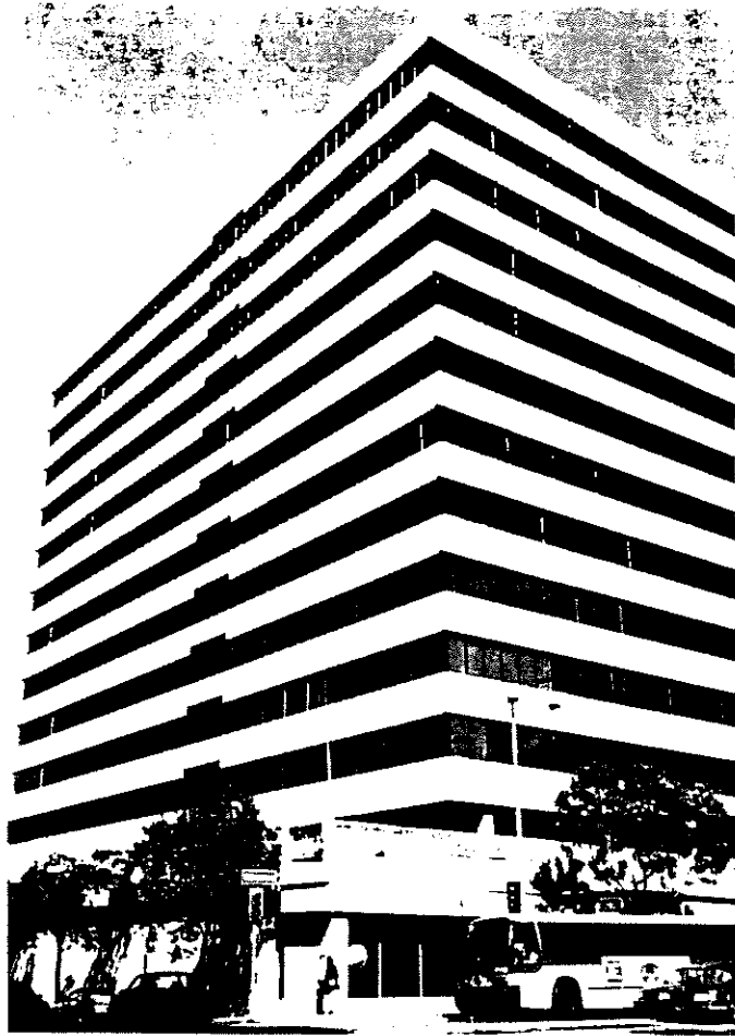
OFFICE TOWER — LOOKING TO NORTHEAST
