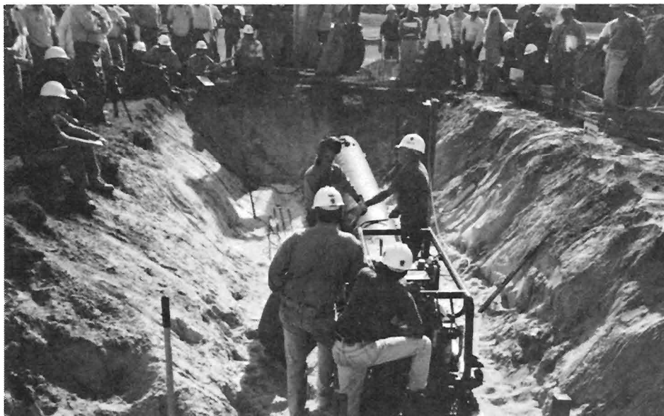
FIGURE 9 Actual field setup of the track type auger boring method.
