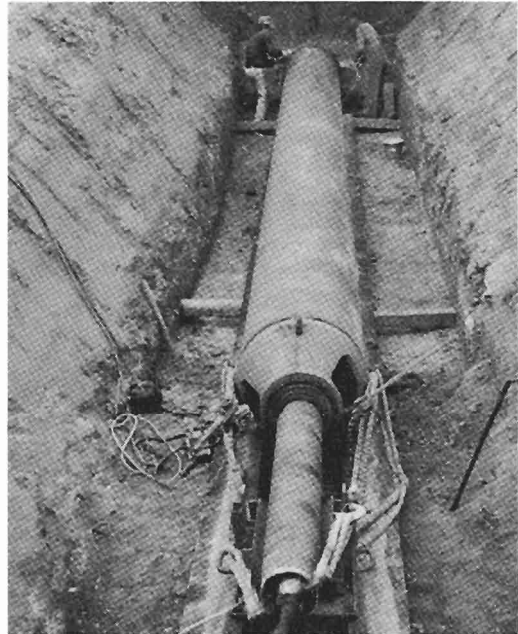
FIGURE 26 Typical field setup for pipe ramming method.
