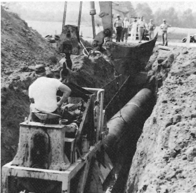
FIGURE 11 Actual field setup of the cradle type auger boring method.
