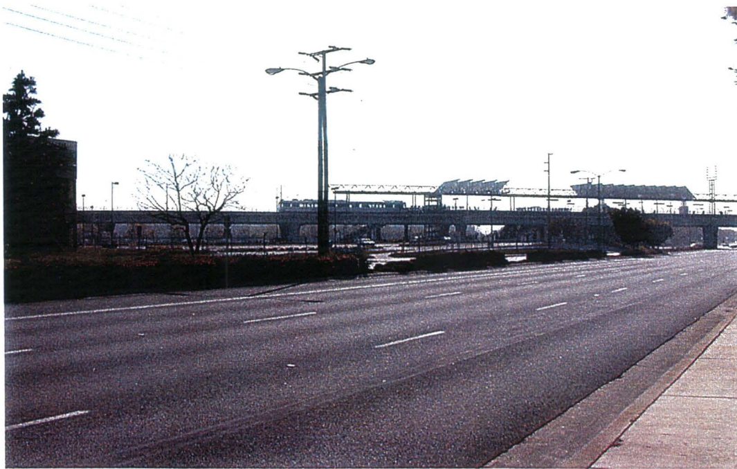
B64: View of the El Segundo Green Line Station parking lot, facing westbound on EL Segundo. Area is light industrial with some outdoor advertisements.
