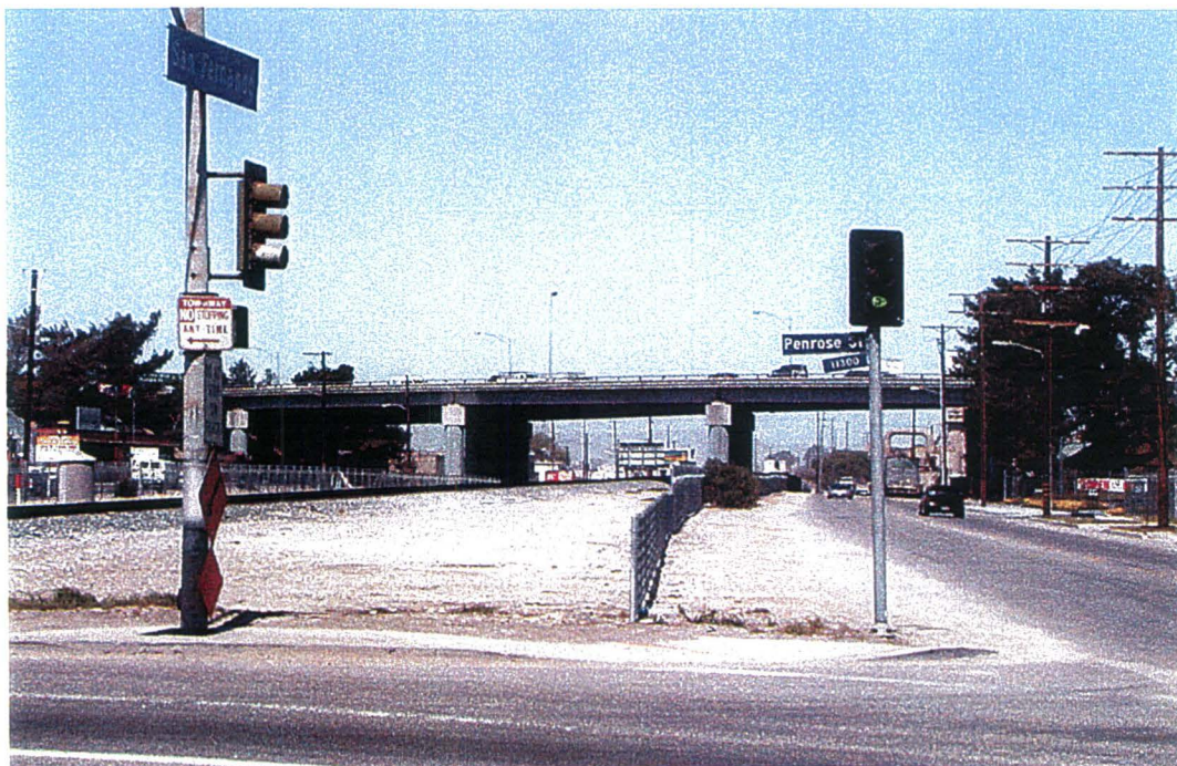
B21: View looking northbound along the MTA right-of-way towards Tuxford Street and the I-5 Freeway overcrossing. San Fernando Boulevard runs parallel to the tracks on the east (right).
