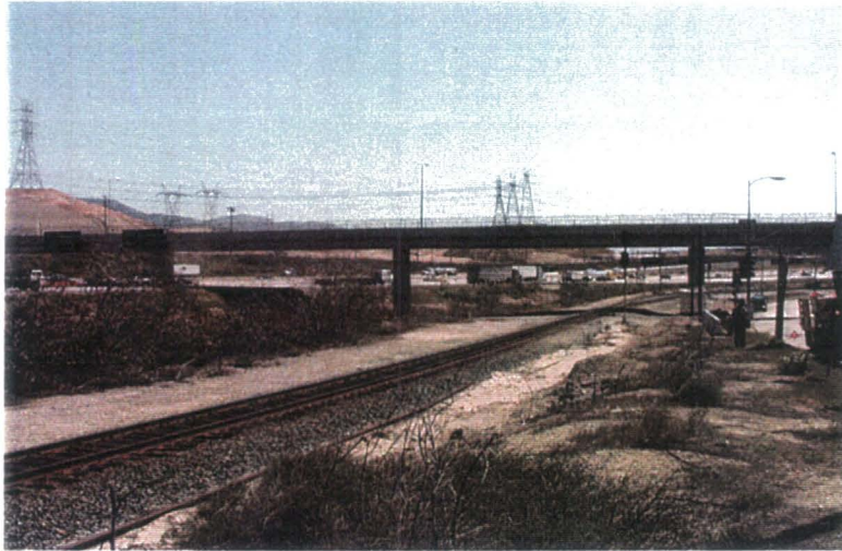
B12: View looking southeast along the railroad right-of-way towards Balboa Boulevard. The site is located on the other side of the bridge. San Fernando Road is seen on the right and the I-5 Freeway on the left. The area contains minimal development. On the other side of the I-5 Freeway there are new industrial park developments.
