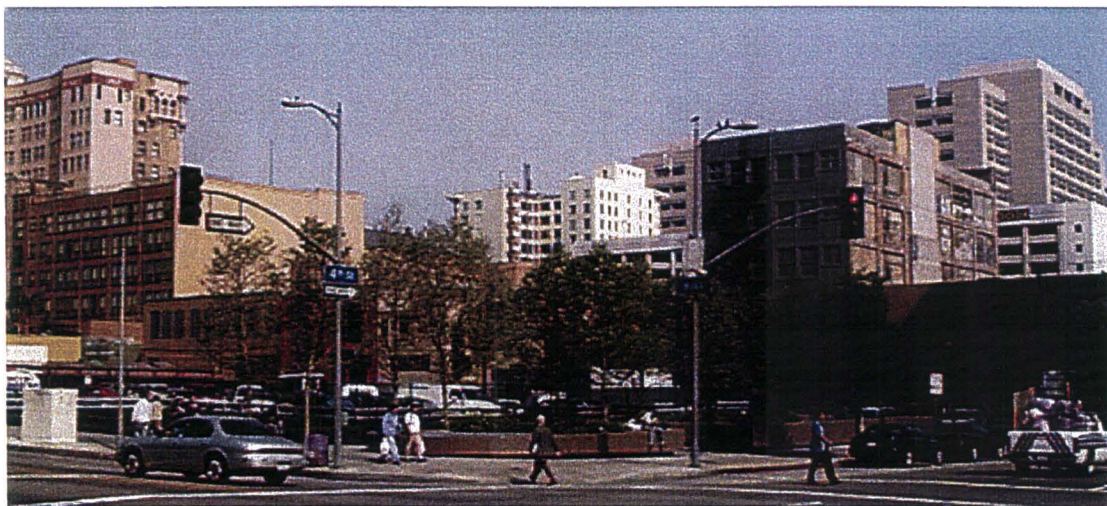
K17: View of the north entrance of the Red Line Pershing Square Station at the northeast corner of Fourth Street and Hill Street.
