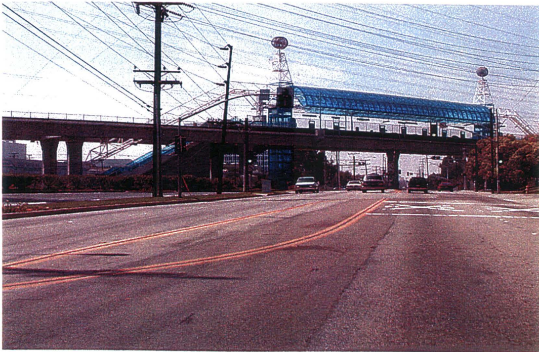
B66: View is looking westbound on Marine Avenue, east of Redondo Beach Avenue. Area is heavily developed with office and light industrial and railroad right-of-way is a prominent feature in the area.
