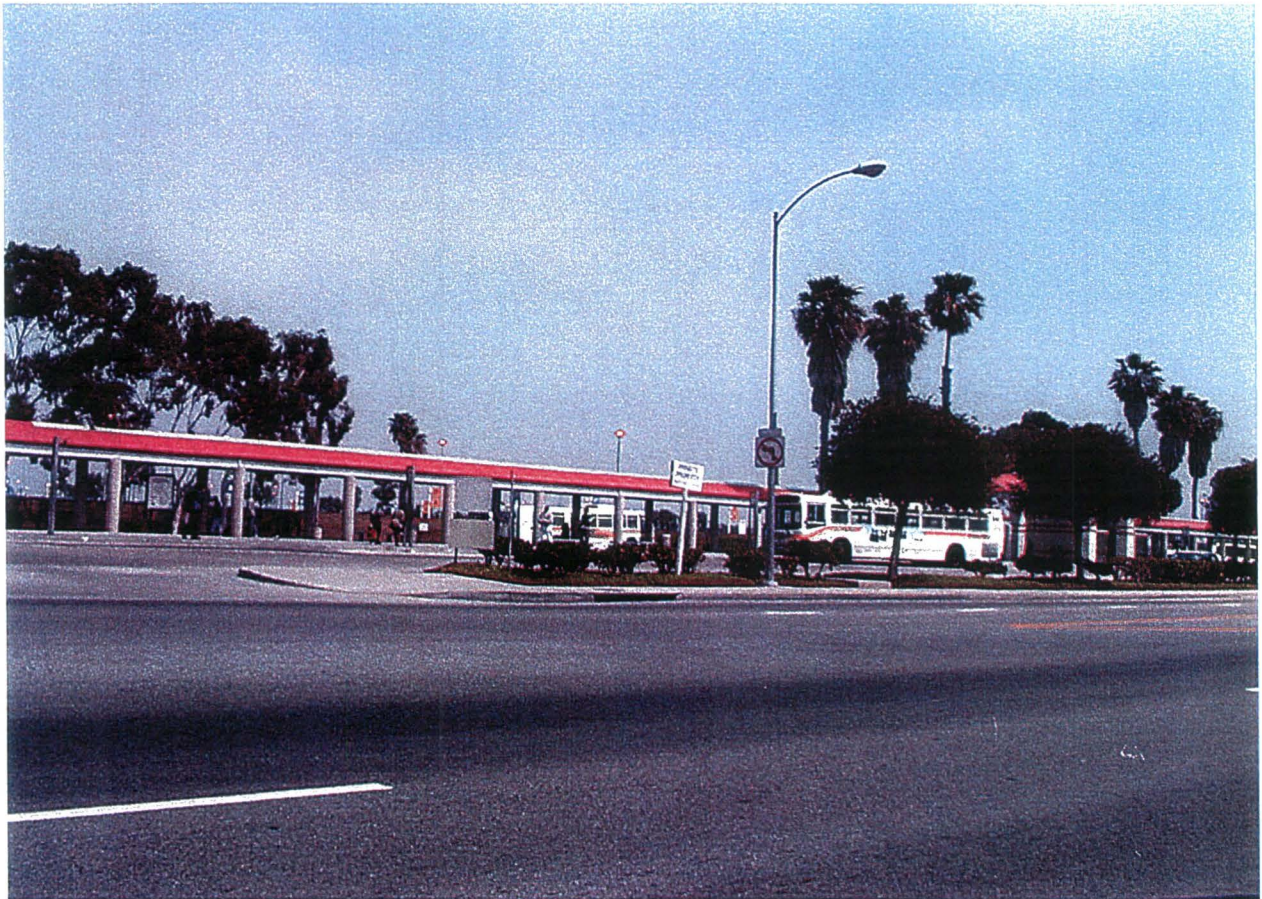
K22 and T8: View of the LAX Bus Terminal facing north from 96th Street. The area consists of rental car lots and airport parking.
