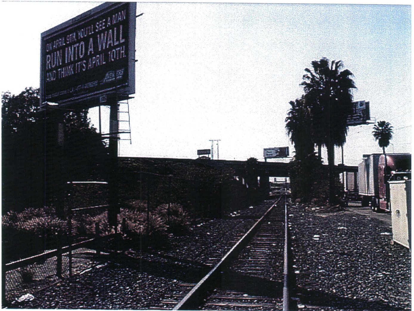
B60: View looking westbound towards the I-5 Freeway overcrossing just south of Slauson Avenue. Area is surrounded by industrial and commercial uses. As shown, several billboards occur in this area.
