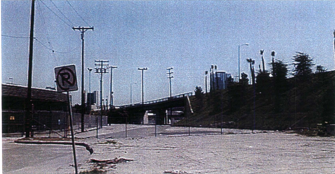
B84: View of Division 12, where the I-710 crosses the Los Angeles River Channel, south of Anaheim Street. Area is comprised of light industrial and residential uses. A few billboards are located in this general area.
