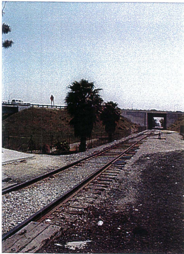
B77: View looking southeast towards the southbound lane of the I-605, just south of the CA-91 interchange. Area is suburban and developed with commercial uses. Billboards are located within this general area.
