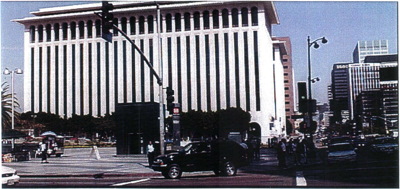
T3 and K11: View of the Red Line Wilshire and Western Metro Station located at the northeast corner of Wilshire Boulevard and Western Avenue.
