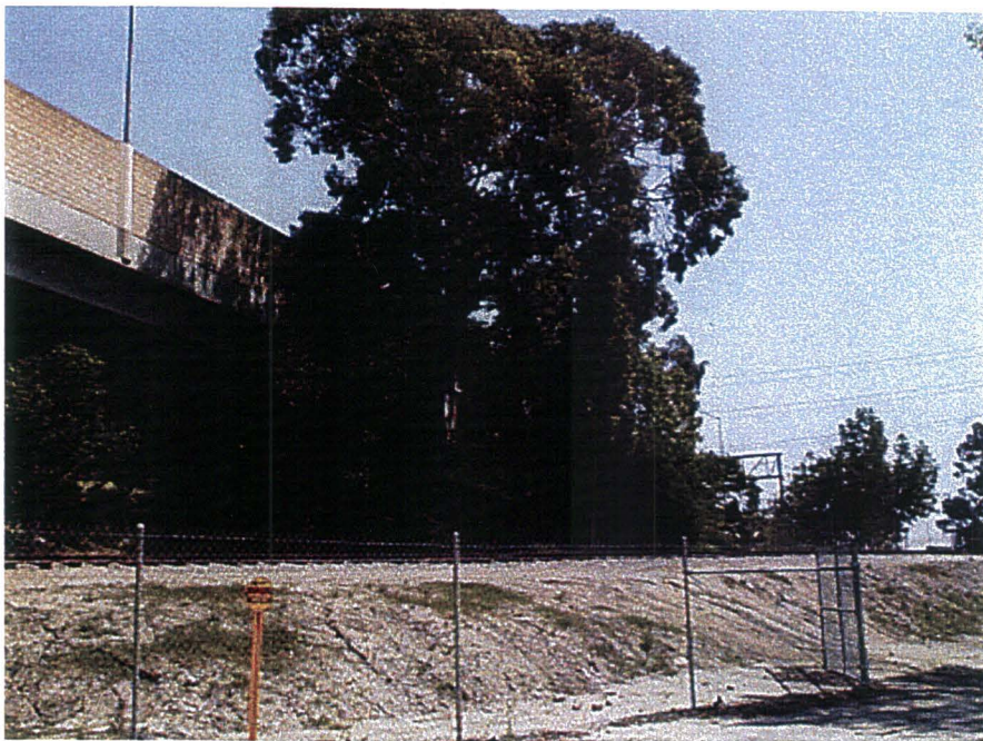
B76: View looking eastbound along the CA-91 Freeway overpass at the Railroad easement. Surrounding area is suburban with nearby residential uses and neighborhood park facilities. No billboards are visible within proximity to this site.
