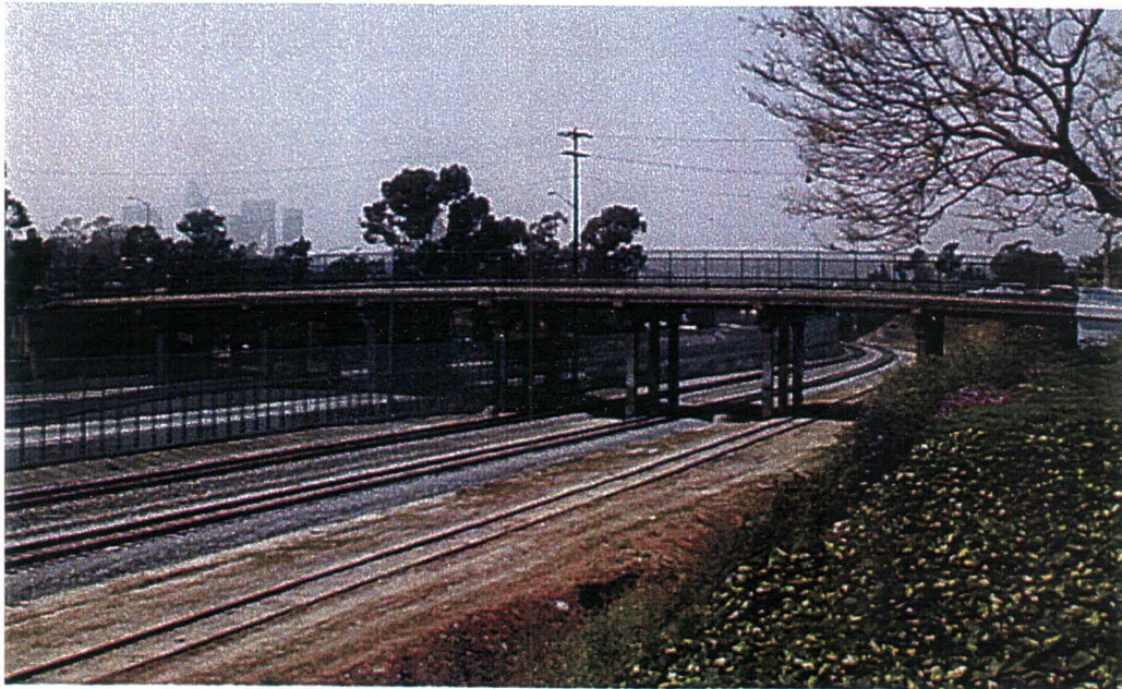
B44: View looking westbound along the railroad right-of-way, parallel to the I-10 Freeway at the State Street overcrossing. Area is developed with commercial, industrial, and high density residential uses.
