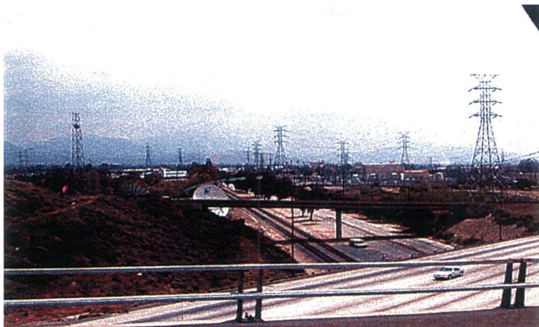
B15: View from the westbound 210 Freeway connector ramp to the southbound I-5 Freeway, looking southeast. Sepulveda Boulevard runs parallel to the MTA right-of-way on the right. The I-5 northbound / 210 eastbound connector ramp is seen below.
