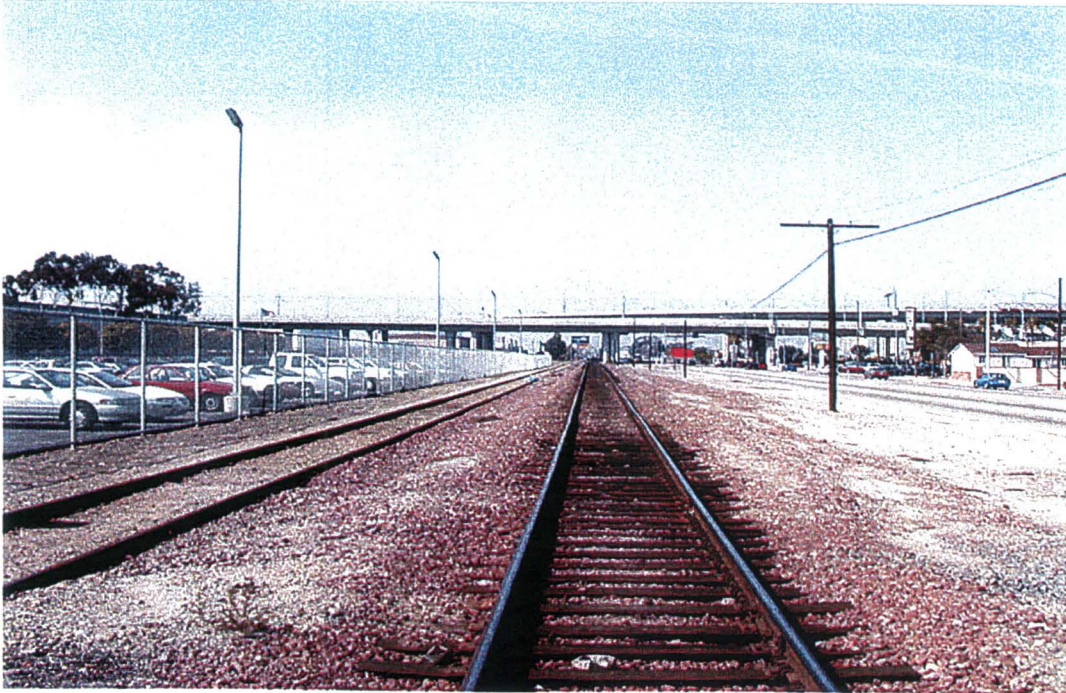
B63: View looking north from 118th Street. Aviation Boulevard is to the east (right) of the tracks. LAX parking is seen to the west (left). The area to the right is residential with some commercial uses. There are billboards and outdoor advertisements in the area.
