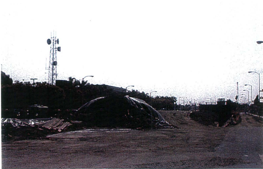
B70: View looking west along Imperial Highway. The MTA police vehicle yard and portable trailer offices are located along the south side of Imperial Highway. Multi-family residential and commercial uses are located along the north side of Imperial Highway in this vicinity.
