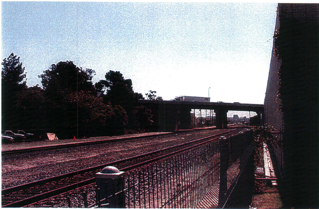
B27: View facing southeast along the MTA right-of-way, towards the I-5 Freeway. The area consists of light-industrial uses and recycling and salvage yards.
