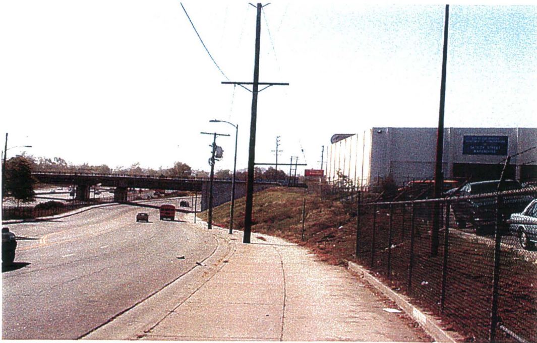
B22: View looking south on Whitsett Avenue. The MTA crossing is seen in the background. The 170 Freeway is to the west (right). A Department of Transportation building is to the east (left). The area is composed of light-industrial land uses.
