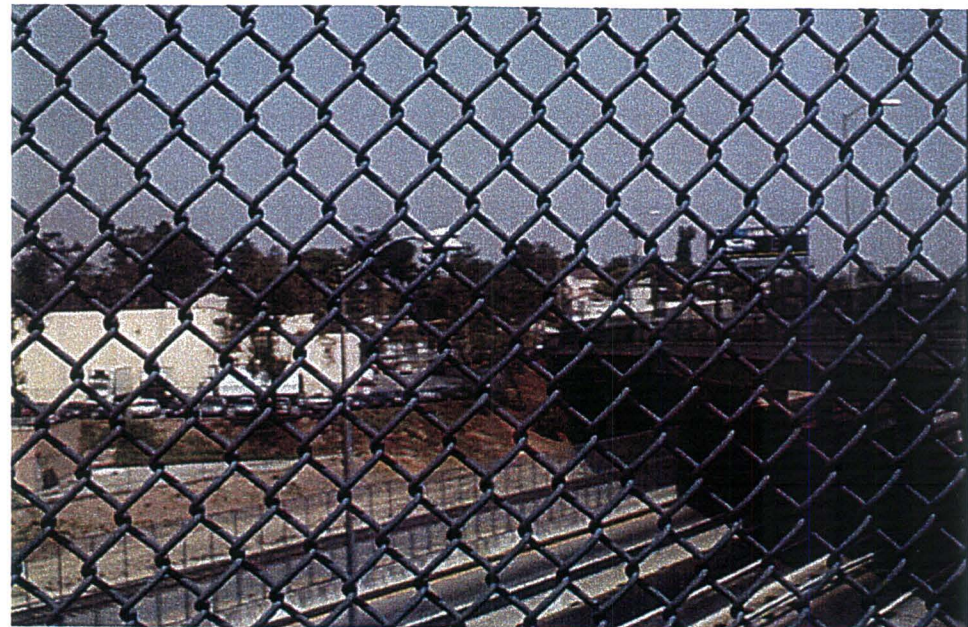
B47: View looking over the I-10 and Soto Street overcrossing from Marengo Street. Area is developed with commercial and high-density residential uses. Numerous billboards are located in the vicinity.
