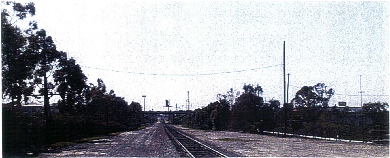
B80: View looking east towards the northbound lane of the I-110 Freeway overcrossing the railroad right-of-way. Area is developed with commercial and light industrial uses. Numerous billboards are visible along the I-110 corridor in this area.
