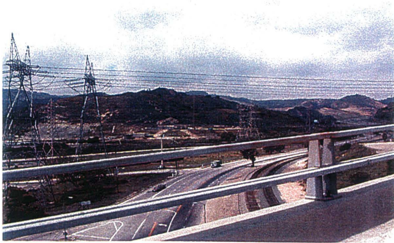
B14: View looking northwest along the MTA right-of-way towards Balboa Boulevard, from the 210 westbound connector to the southbound I-5 Freeway. San Fernando Road is seen on the left.
