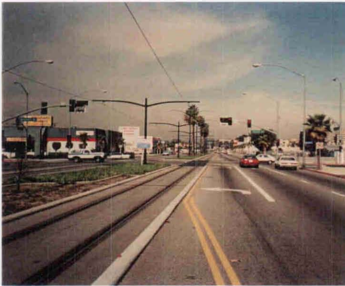
Figure 3-1 SEPARATE TRAFFIC LANE AND SIGNAL PHASE FOR TRAFFIC TURNING LEFT FROM STREET RUNNING PARALLEL TO LRT TRACKS
