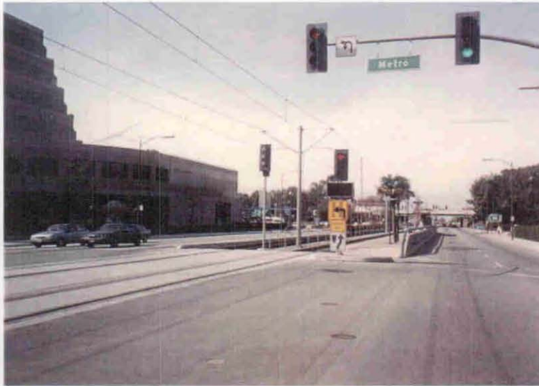
Figure 3-3 TRAIN-ACTIVATED WARNING SIGN FOR TRAFFIC TURNING LEFT FROM STREET RUNNING PARALLEL TO LRT TRACKS
