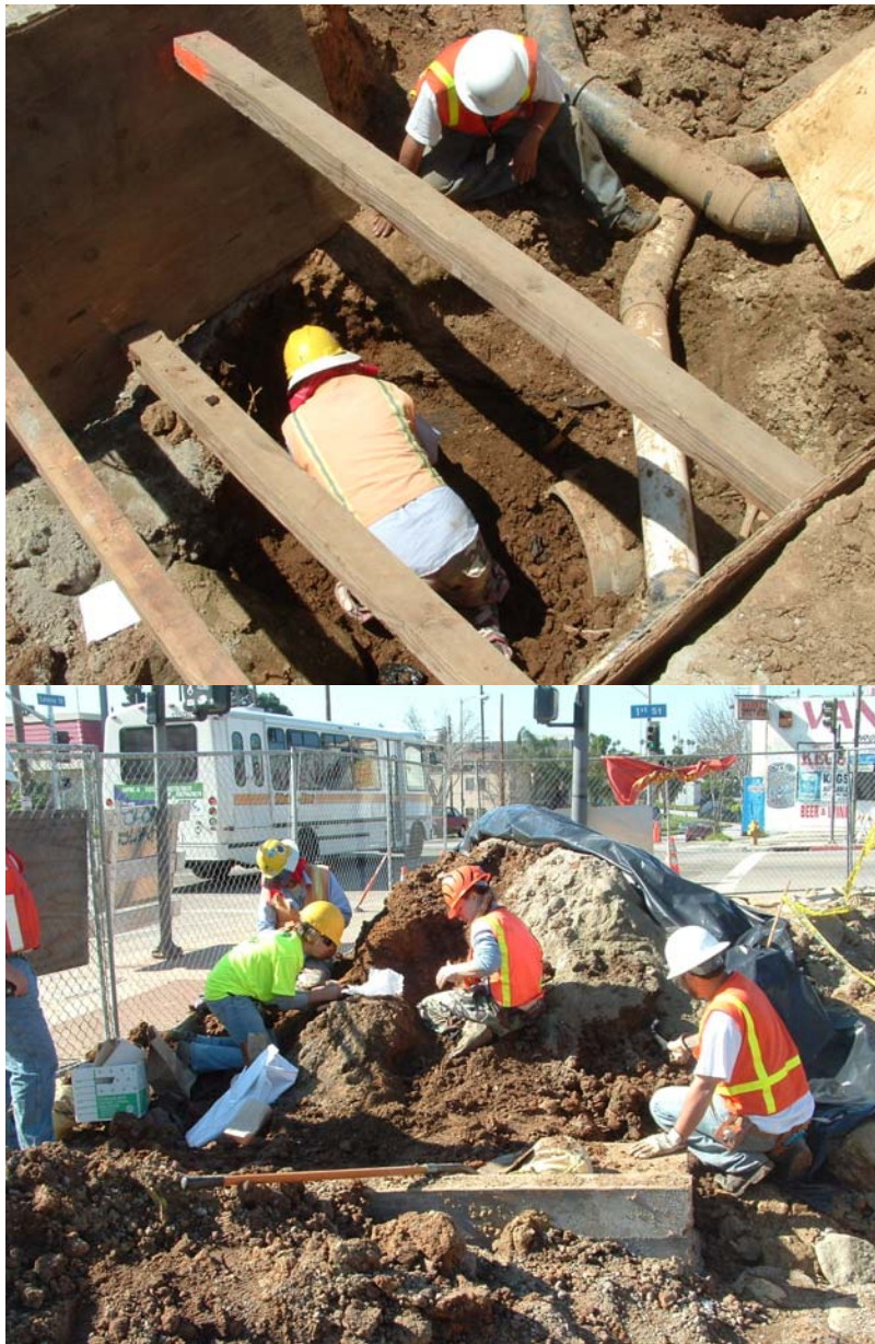
Figure 2.6. Excavation of recovery in the pipe trench and stockpile exploration
