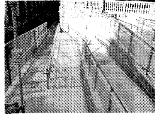
Memorial Park (complex ramps and narrow entry leave no space for gates)
