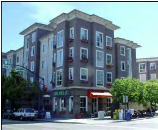
Illustrative Photo: Four-story mixed-use buildings
