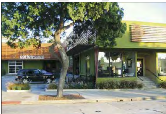
Example: Commercial building with parking on the side and buffered by landscape
