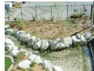
Storm water treatment
