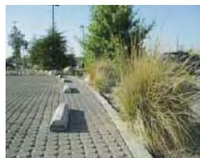
Permeable paving for parking
