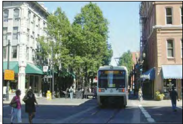
Illustrative Photo: Four story mixed-use buildings
