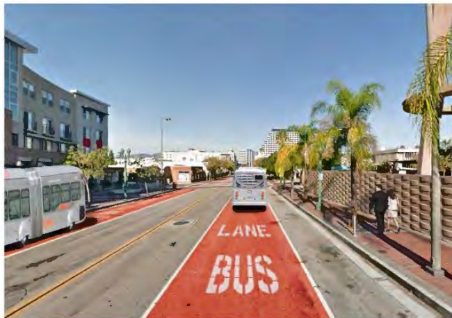
Side-Running Dedicated BRT Lanes on Broadway, West of Glendale Boulevard, in Glendale
