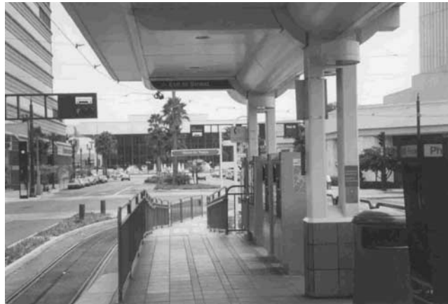
Figure 5-9: TVMs on Platform at Los Angeles Blue Line Station
