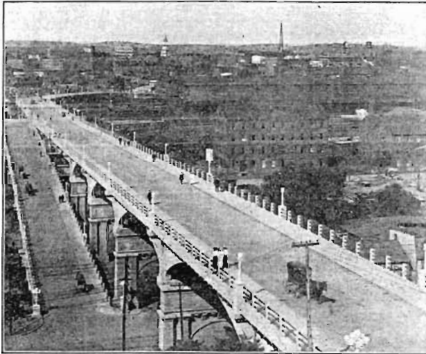
ARTISTIC ELEVATED STREETS. Mulberry Street Bridge, Showing Incline.
