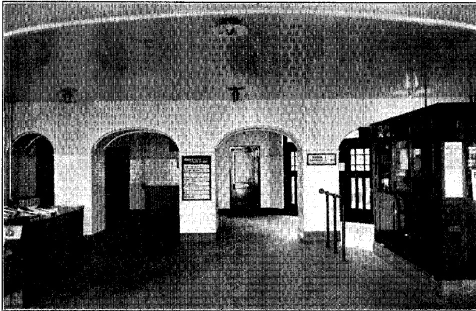
FIGURE 53. Interior of station on the Northwestern Elevated Railway in Chicago.
