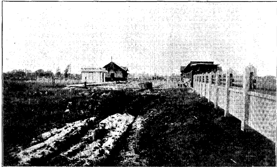
FIGURE 57. Vicinity of Lawrence and Kimball Avenues, Chicago, before elevated railroad construction.
