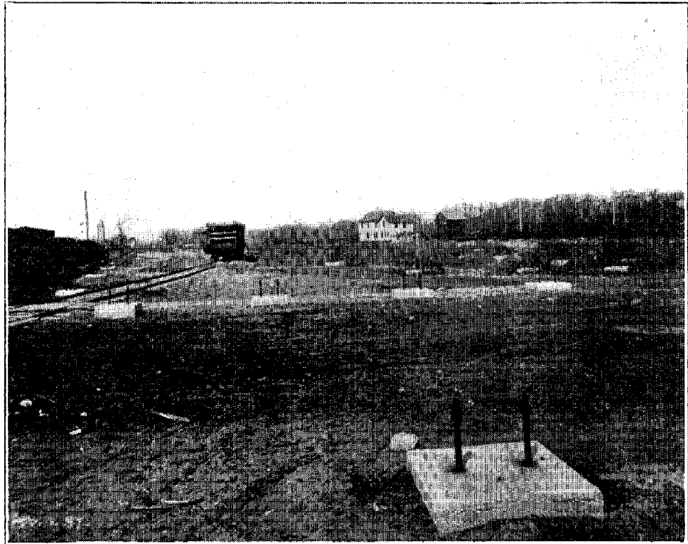
FIGURE 59. Vicinity of Broadway and Wilson Avenue, Chicago, before elevated railroad construction.
