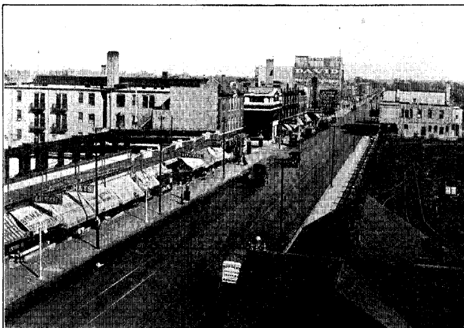
FIGURE 58. Vicinity of Lawrence and Kimball Avenues, Chicago, after elevated railroad construction.
