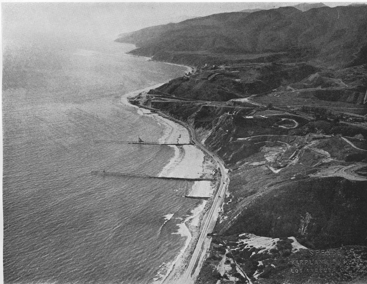
PLATE 37. Beach above Santa Monica that would be inside proposed harbor, showing groins built far out on the beach to protect the shore and catch the drifting sands. (Photo by Spence.)
