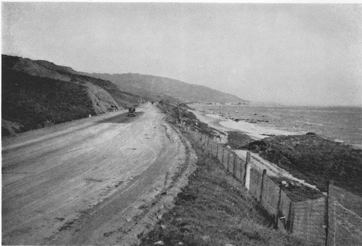
PLATE 3. New highway along the ocean front, showing narrow strip of private lands fenced in and cutting off all access to the publicly owned tidelands.
