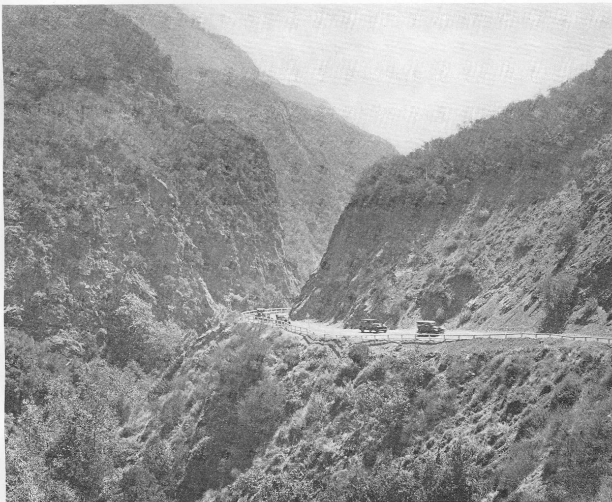
PLATE 50. Rugged and picturesque cliffs along Lower Topanga Canyon, where land has little value for houses and should be preserved for scenery. (Photo by Stagg.)
