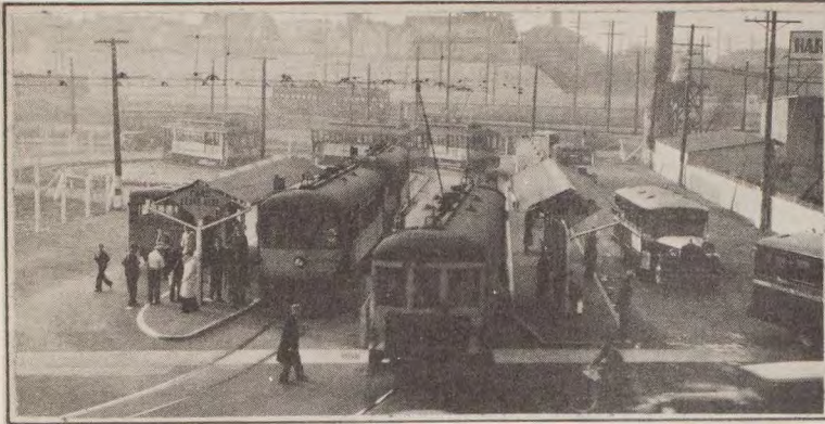
Street Car and Motor Coach Terminal at Pico and Rimpau Loop System for All Operations providing for off-street facilities
