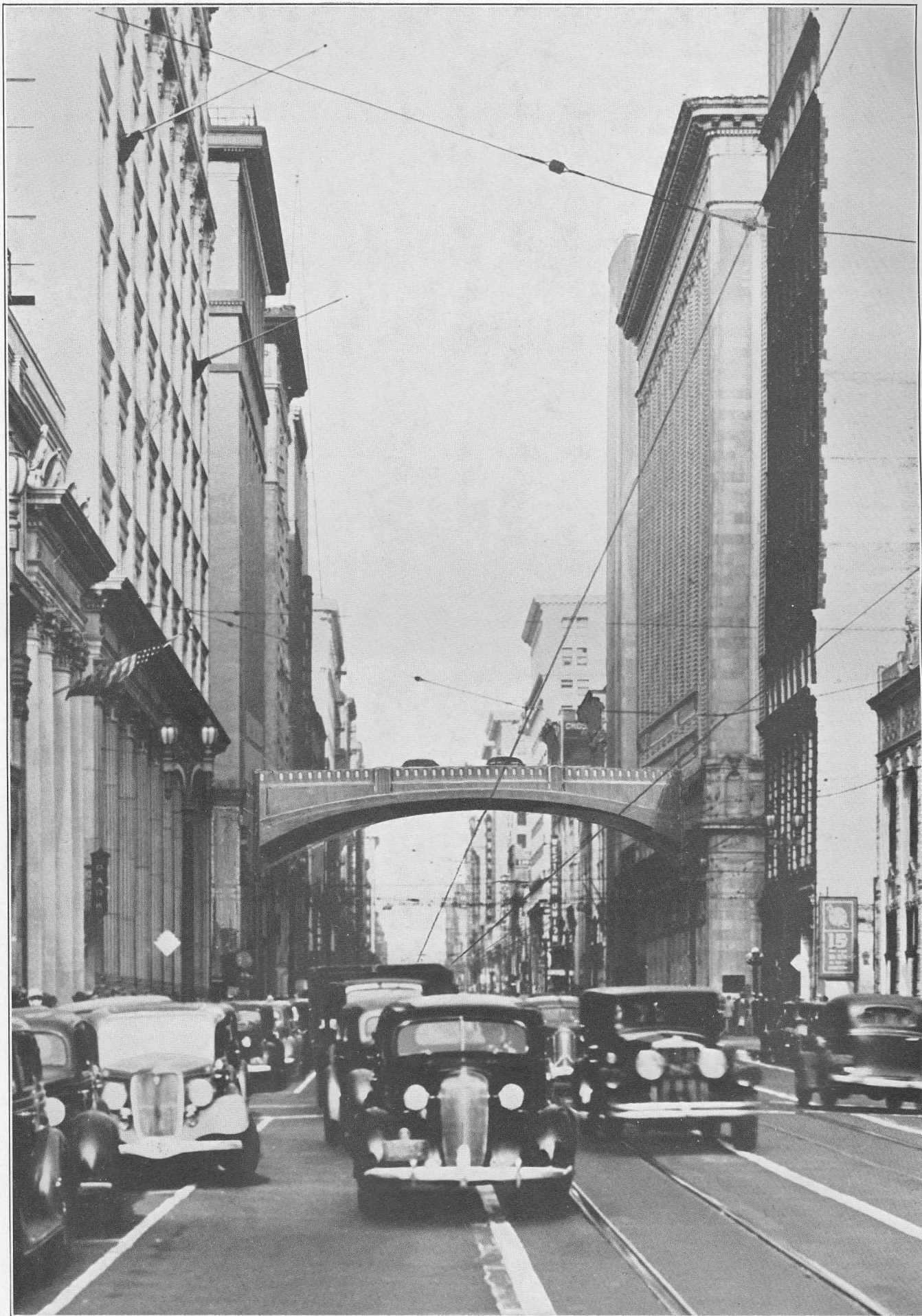
COMPOSITE PHOTOGRAPH—MOTORWAY BRIDGE OVER TYPICAL COMMERCIAL STREET
