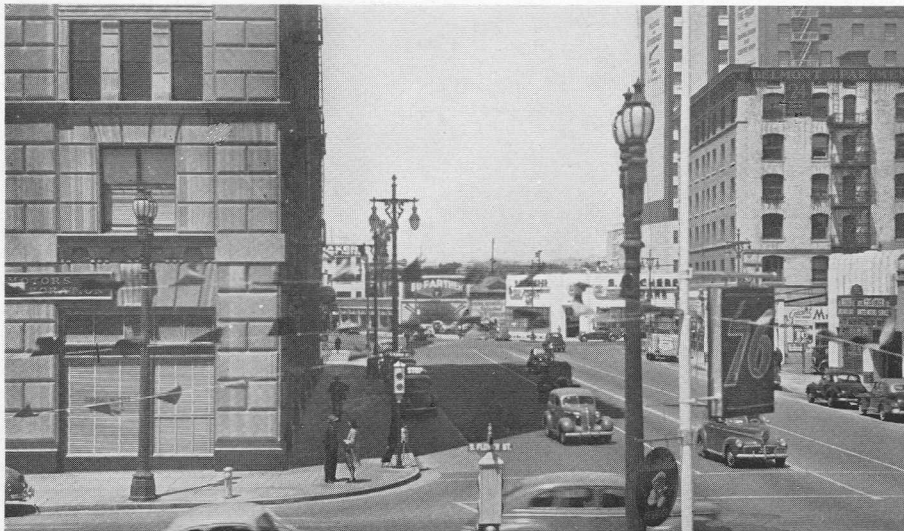
Olympic Boulevard and Flower Street, 1941, the Widening Job Completed
