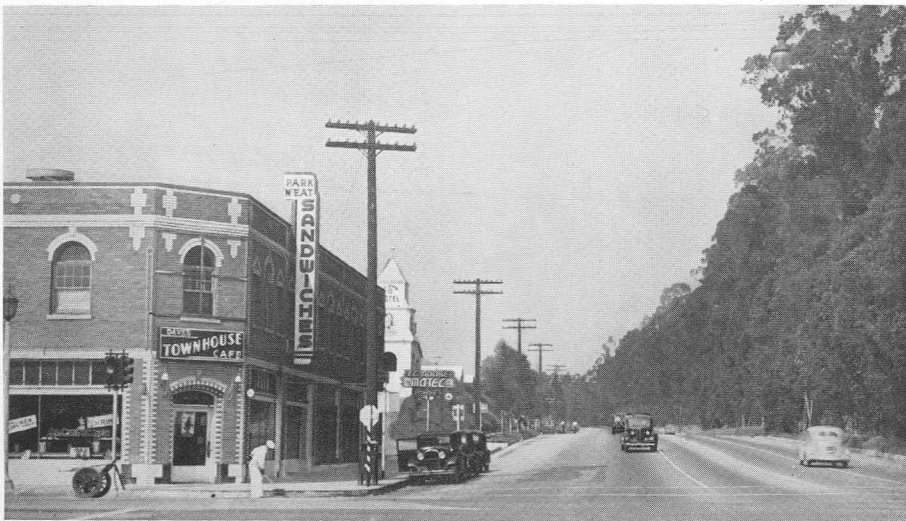
Garvey Avenue at Atlantic Boulevard, 1941, Small Land Cost for Widening
