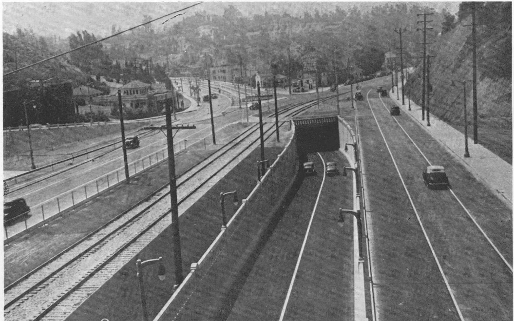
Slot Type Intersection on Cahuenga Freeway
