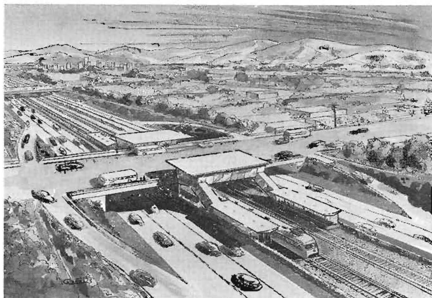
Typical station... Surface transit will feed rail rapid transit for fast operation.
