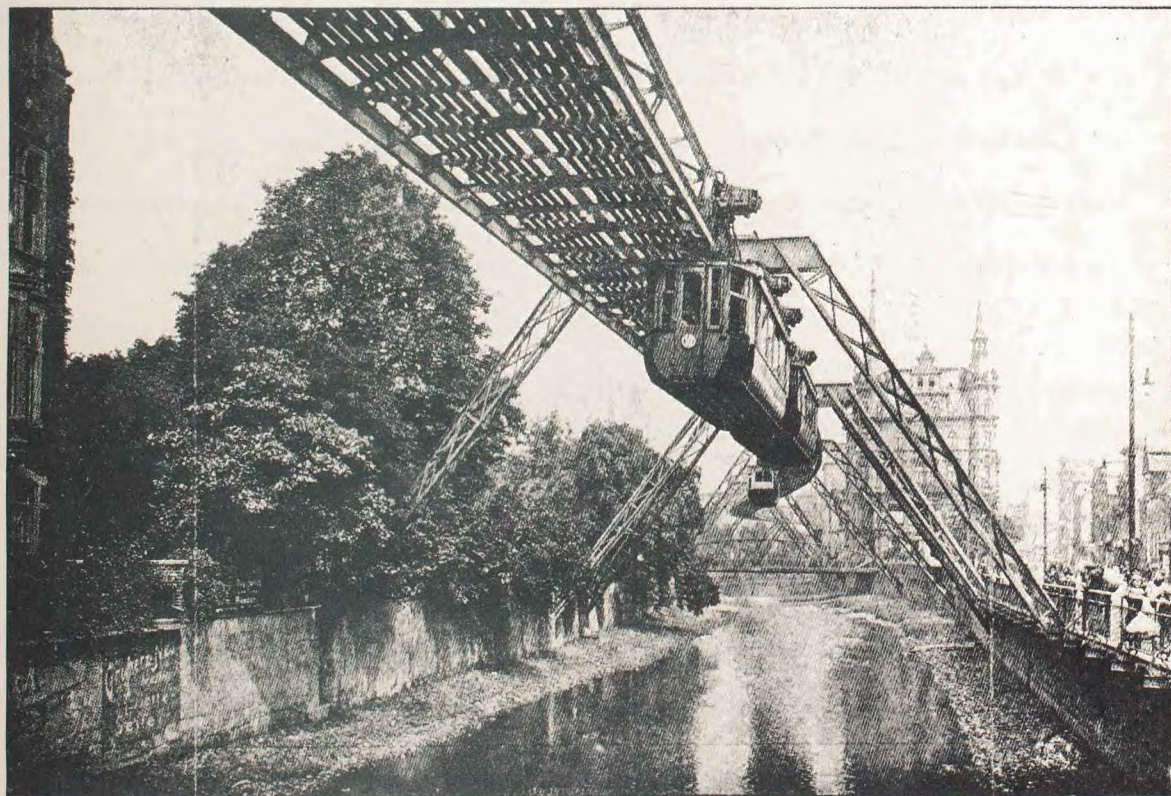
Barmen-Elberfeld-Vohwinkel Suspended Electric Railway. Above the Wupper River in Barmen.
