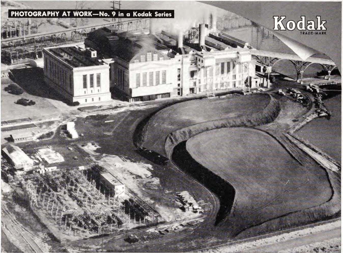
Richmond Station of the Philadelphia Electric Co.
