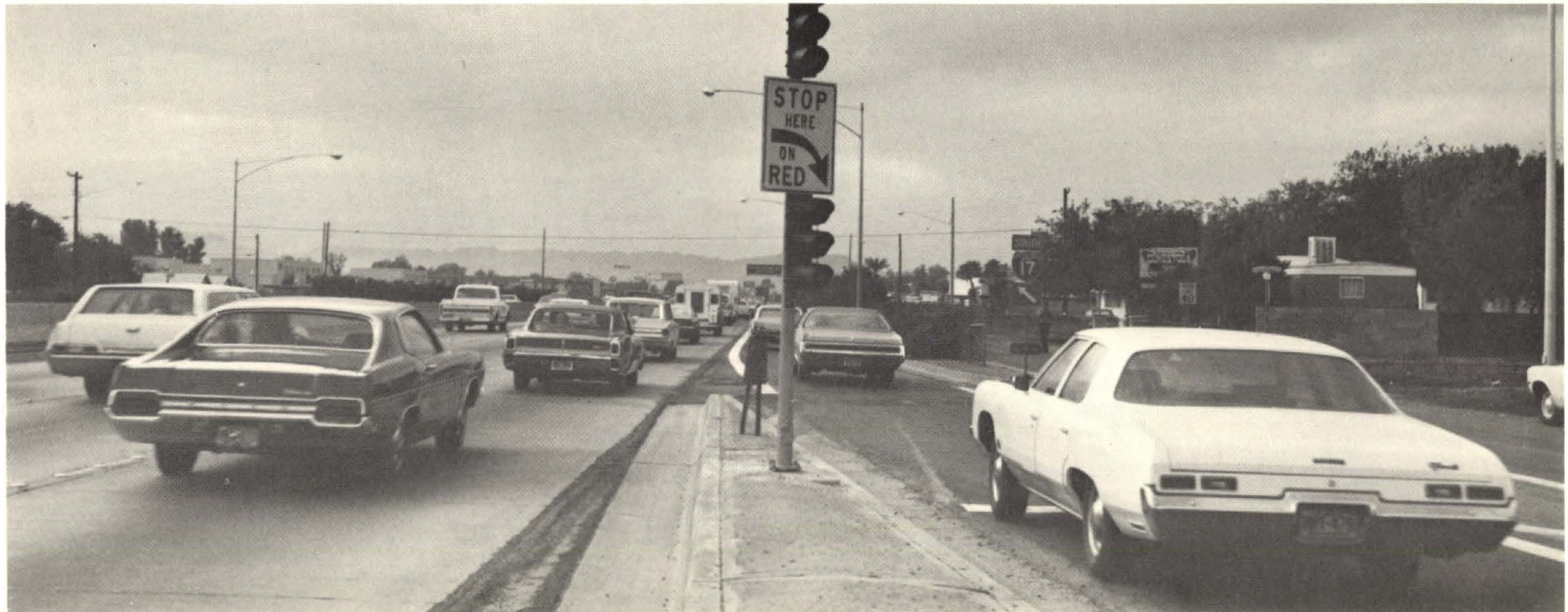
▲ Entrance ramp control is used to reduce the number of vehicles entering the freeway, thus allowing the freeway to move in the most efficient range of speeds and
