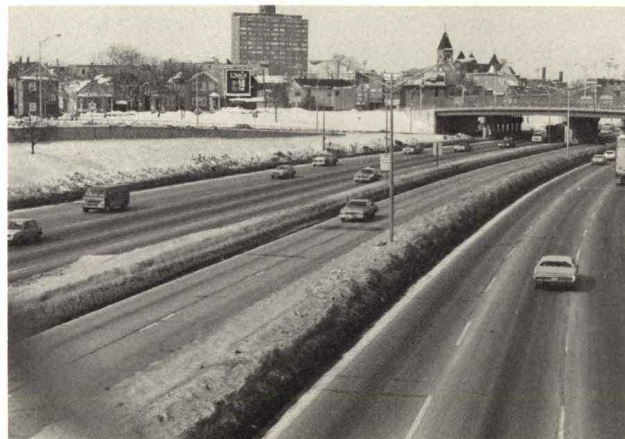
▲ Separated limited access roadways are constructed for the exclusive use of high-occupancy vehicles. (Chicago Regional Office - Alan M. Voorhees & Associates.)
