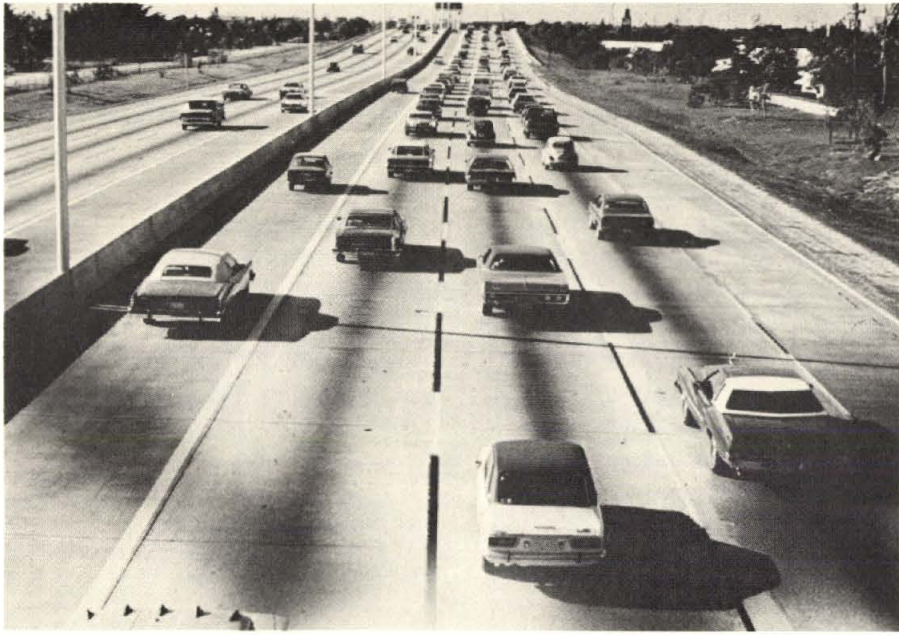
▲ Relatively inexpensive to implement, a concurrent-flow reserved lane gives high-occupancy vehicles a travel time advantage. (Florida Department of Transportation.)
