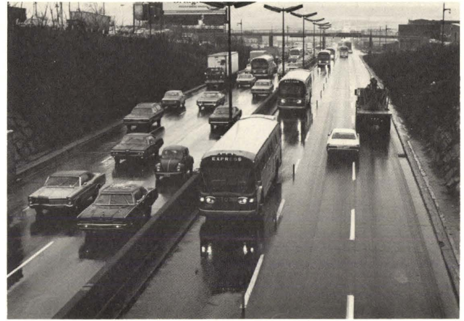
▲ In a relatively short time and at low cost, peak-direction capacity can be increased by the use of contraflow lanes. (The Port Authority of New York and New Jersey.)
