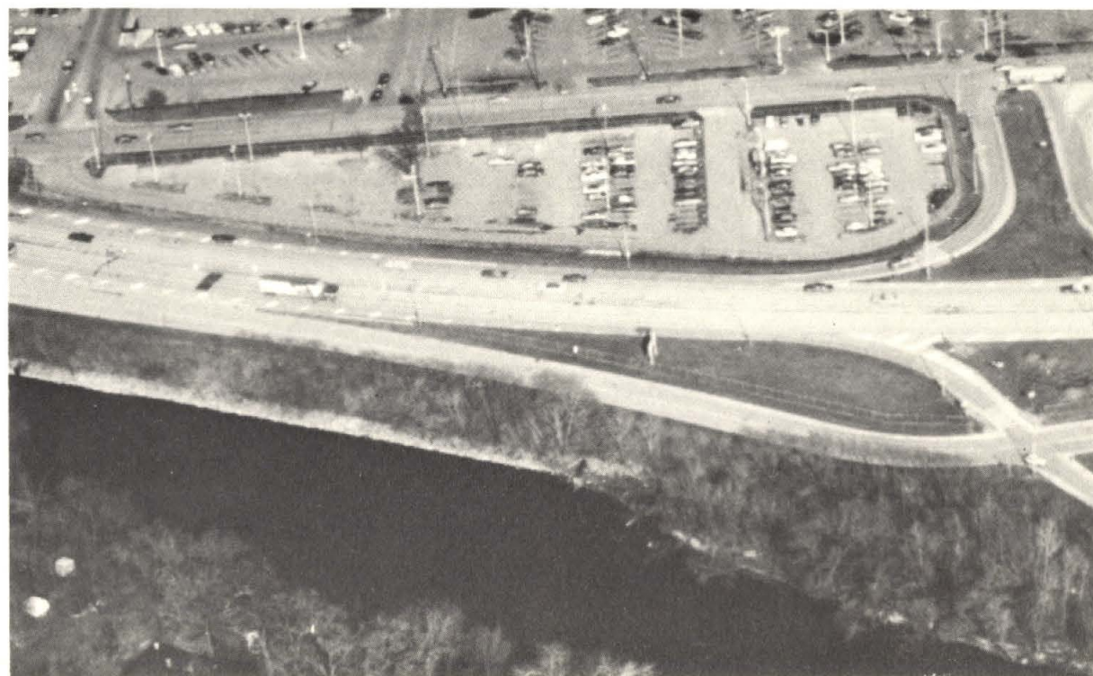
▲ Located at strategic points with easy access to the freeway, park-and-ride facilities can encourage transit use and ridesharing participation by serving as convenient collection points. (California Department of Transportation.)
