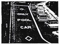
Ramp meter bypass, California
