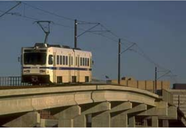
An aerial LRT structure in Baltimore.
