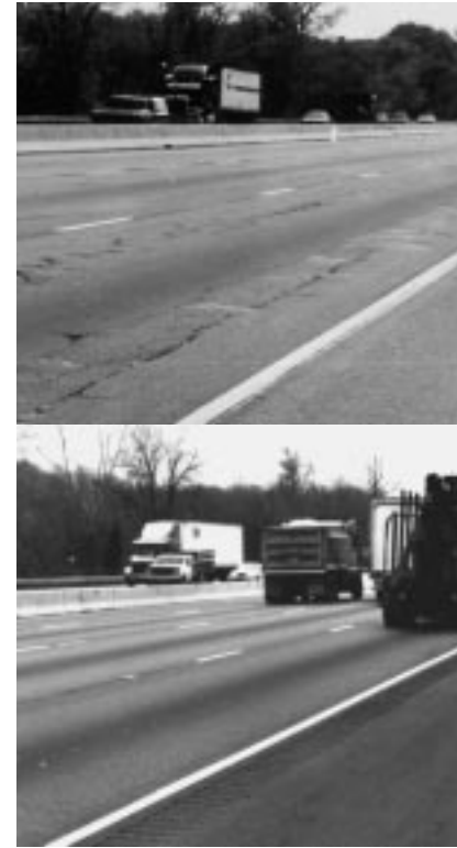
Standing committees have promoted innovative approaches to long-lasting pavements. Perpetual asphalt paving is an example: in 1993, after 26 years of service, New Jersey I-287 appeared to be in terminal condition (top); the top 4 inches of surface were replaced and the roadway remained in good condition 7 years later (bottom).
