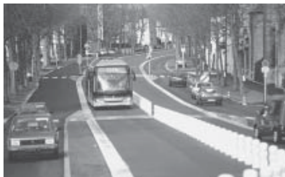
Bus rapid transit vehicles, the subject of TCRP Report 90, Volume 1, Bus Rapid Transit: Case Studies in Bus Rapid Transit , operate primarily in fast and easily identifiable exclusive transitways or dedicated bus lanes.
