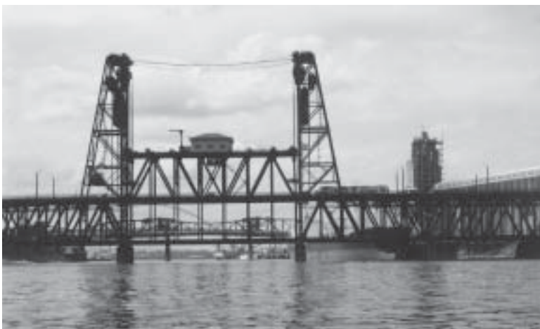
Terminal ( top ) and lift bridge in the Port of Portland, which several committees toured during a joint midyear meeting.
