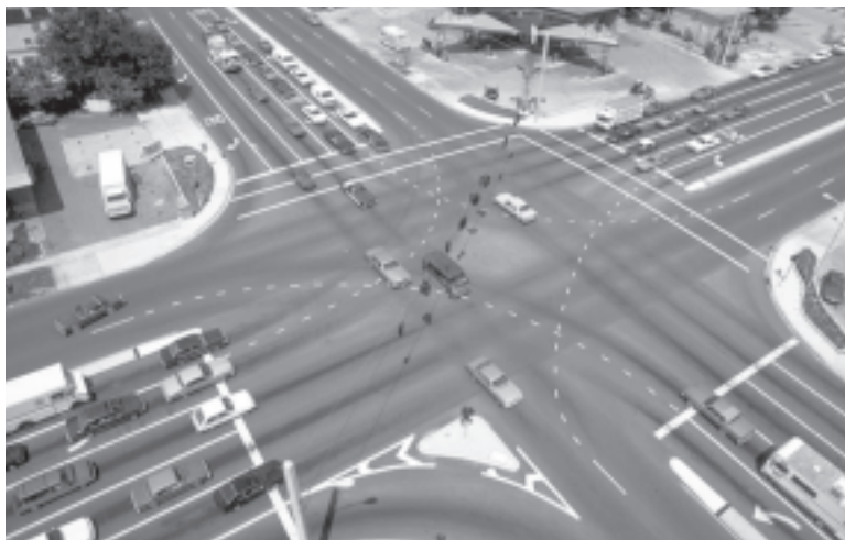
Delineation of turn paths for double left-turn lanes is included in research for NCHRP Report 500, Volume 12, A Guide for Reducing Collisions at Signalized Intersections .
