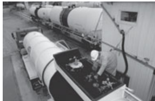
Hazardous materials transportation research under HMCRRP will involve multimodal and intermodal issues. Photo shows the transfer of hazardous materials from a tanker truck to a rail car.
