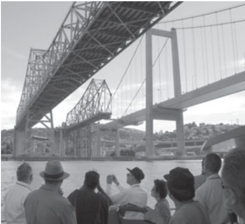
The Fifth National Seismic Conference on Bridges and Highways included a tour of bridges and bridge construction in the San Francisco Bay Area; (above) the old Carquinez Bridge, under demolition, with the new suspension bridge in the background.
