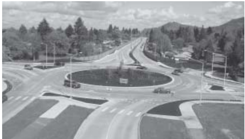
The safety and operational effects of roundabouts—like this in Springfield, Oregon—are the subject of NCHRP Report 572, which includes updated design criteria.
